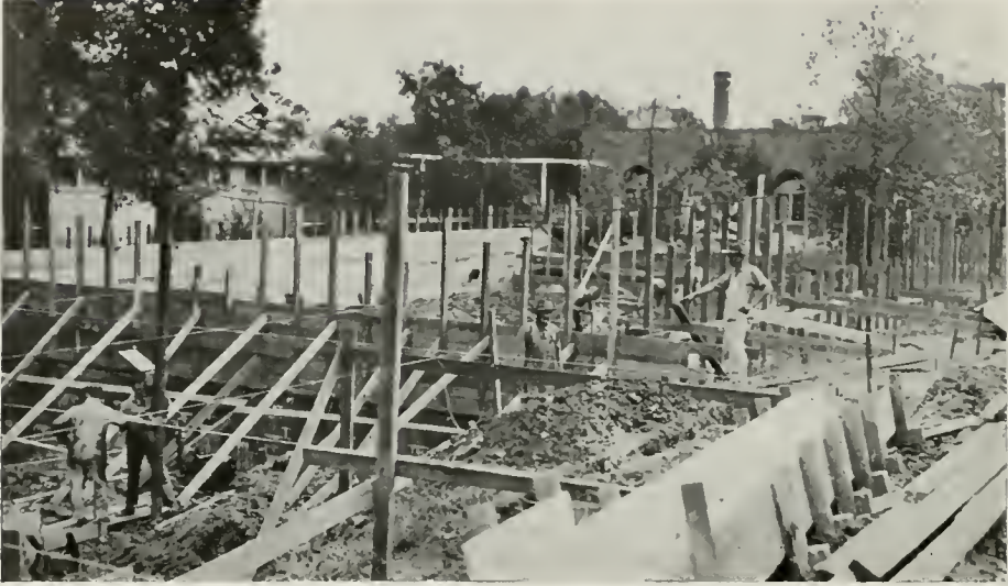
SWIMMING POOL DURING CONSTRUCTION
