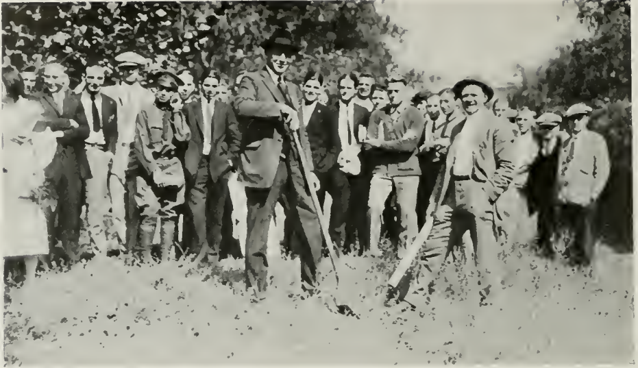
BREAKING GROUND FOR THE SWIMMING POOL
