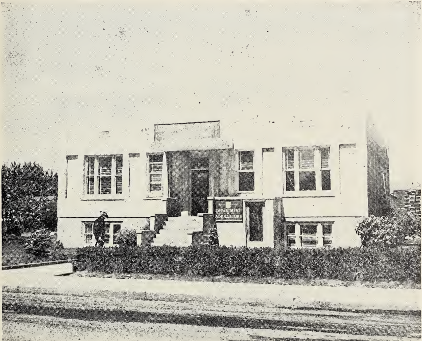
OFFICES OF CAMROSE MUNICIPAL DISTRICT NO. 63
