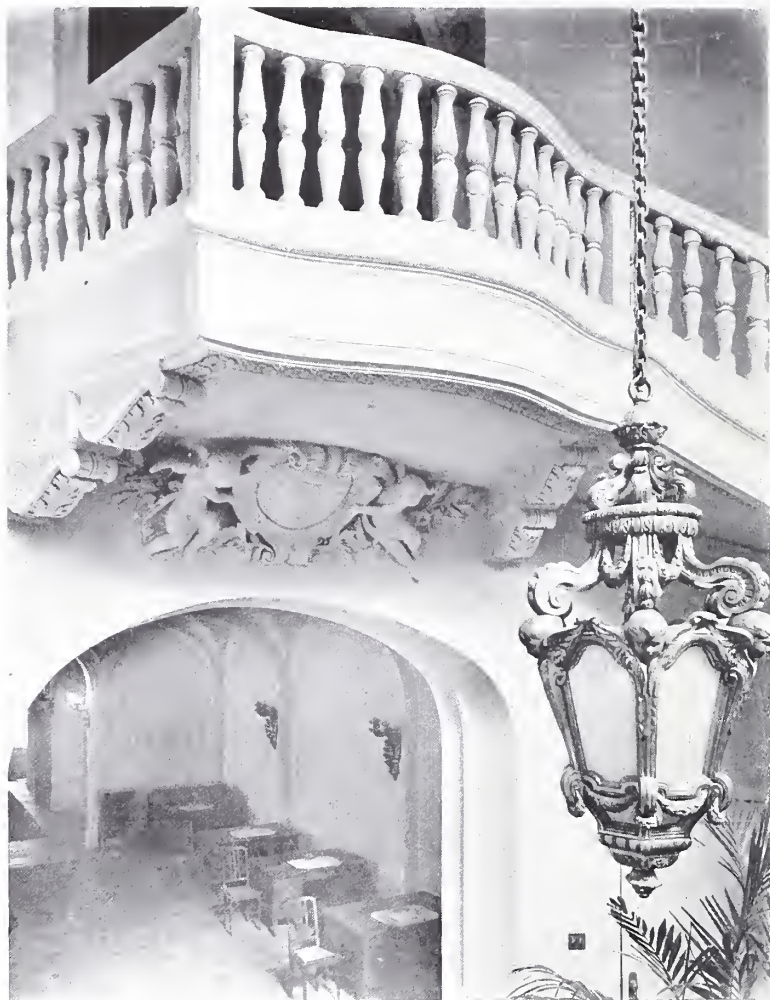
ADAPTED ITALIAN RENAISSANCE IN A COMMERCIAL BUILDING
