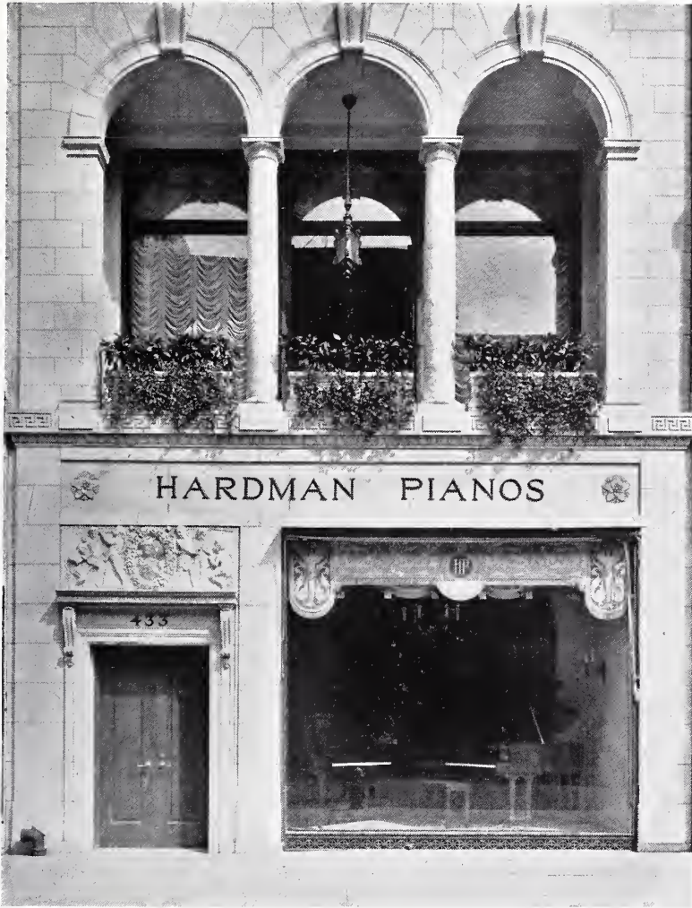
A DETAIL OF THE TWO LOWER STORIES OF A COMMERCIAL BUILDING
