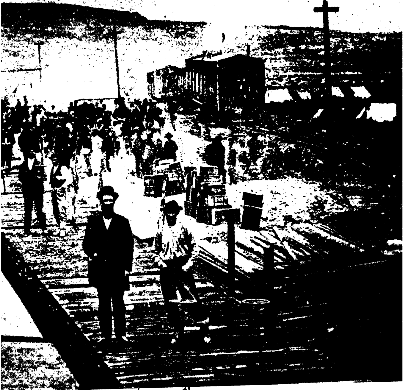
A CHAMPION CREW displays some of the equipment (above) that helped it lay 10 miles of track in a day. This feat won the Central Pacific's construction boss a $10,000 bet from an official of the Union Pacific. The U.P.'s best was eight and a half miles in one day.
