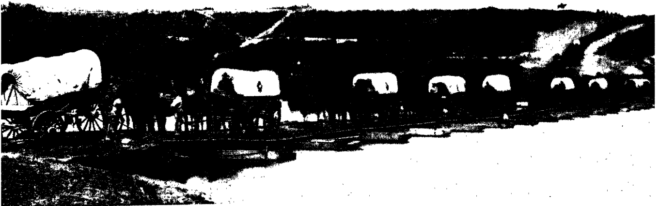
A BRIDGE ON THE RAPPAHANNOCK easily accommodates a long supply train. The pontoons that supported such bridges were square-ended wooden or canvas boats 20 to 30 feet long;
