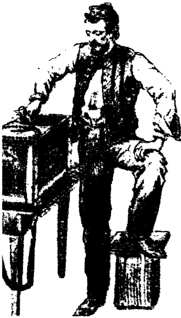
A Union telegrapher sends a message on a machine used by operators who did not know code. When they dialed a letter, a machine at the other end registered the same selection. A rising businessman named Andrew Carnegie helped organize the army telegraphers. Some 40 years later, millionaire Carnegie pensioned more than 100 Civil War telegraphers or their widows.
