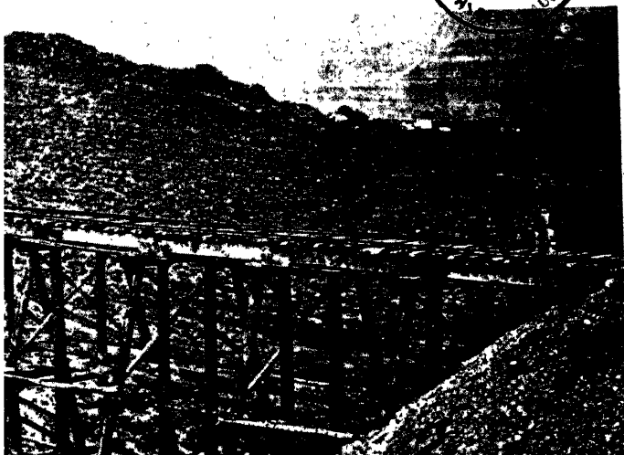
A TEMPORARY TRESTLE, built in six weeks over a 450-foot cut east of Promontory, is crossed by Engine No. 119. The wooden trestles later had to be banked with rocks or replaced with a more durable construction. Promontory was bypassed by a new line in 1904.
