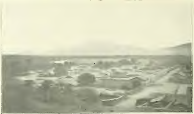
A VIEW OVER THE TOWN OF MORROPÓN, PIURA VALLEY. Note the two bodies of insect-breeding stagnant water. There is much malaria at Morropón.
