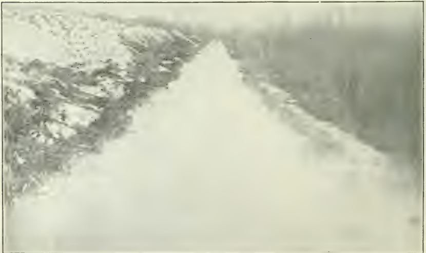
A corresponding view on January 26, 1916, showing where some of the sewage effluent drains enter the stream, as well as the appearance of the banks in winter and the increased volume of water.
