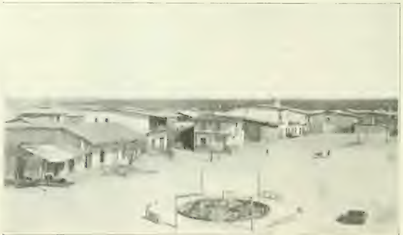
THE PLAZA AT SECHURA, NEAR THE MOUTH OF THE PIURA RIVER.
