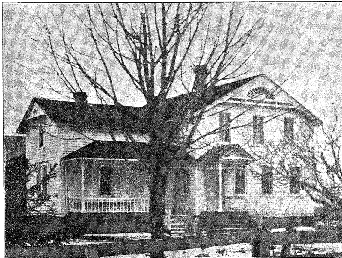
RESIDENCE OF J. P. KORMAN, FRANKENLUST.
