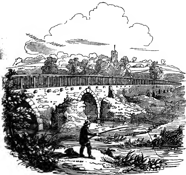
OLNEY BRIDGE, BUCKINGHAMSHIRE.
