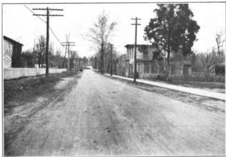
FIG. 2.—MARYLAND STATE HIGHWAY, CONCRETE.
