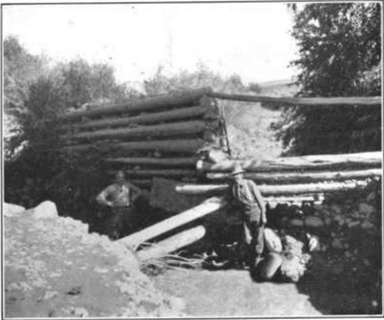
FIG. 1.—IMPORTANT IRRIGATING DITCH AND LATERAL LESS THAN ONE MILE FROM BUSINESS SECTION OF EPHRAIM CITY, UTAH, BADLY DAMAGED BY THE FLOOD OF AUGUST 24, 1912.
