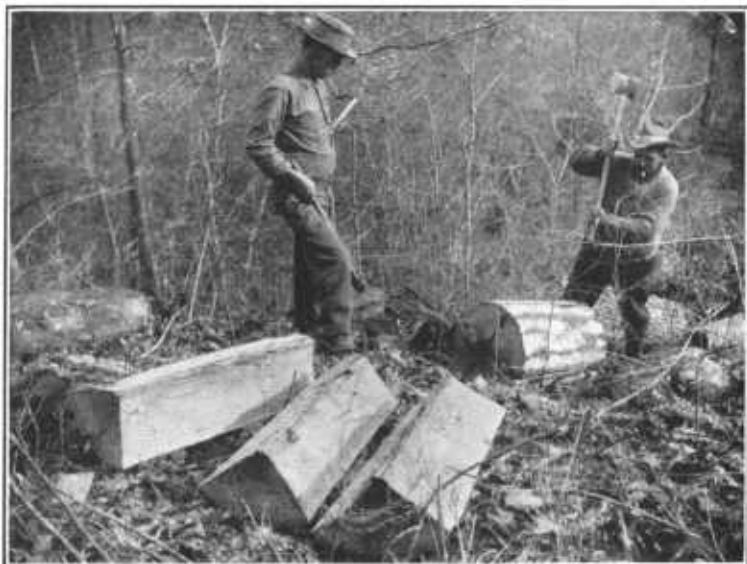
FIG. 1.—QUARTERING STAVE BOLTS ON HOMESTEAD.
