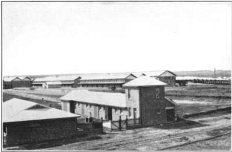
FIG. 2.—GENERAL VIEW OF THE NEW STATE ABATTOIR AT SYDNEY, AUSTRALIA.
