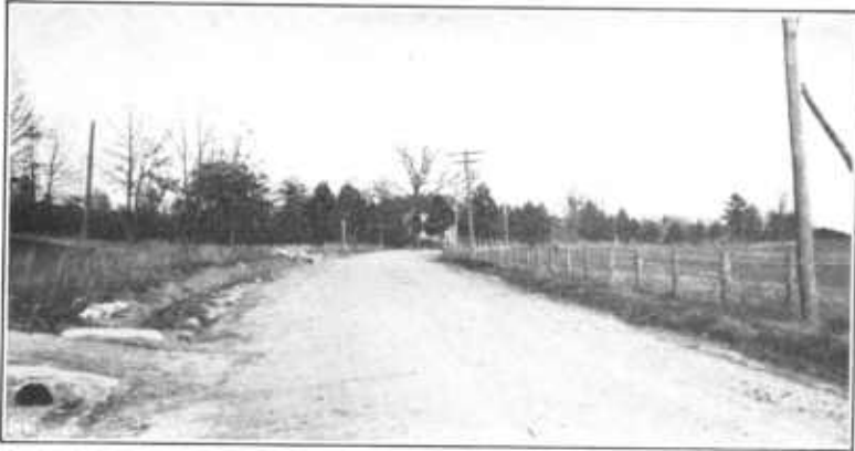
FIG. 1.—VIRGINIA STATE-AID ROAD, TOPSOIL AND GRAVEL.
