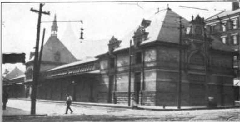
FIG. 3.—PEARL STREET MARKET IN CINCINNATI, AN EXAMPLE OF THE LONG, NARROW TYPE OF MARKET HALL LOCATED IN THE MIDDLE OF THE STREET.
