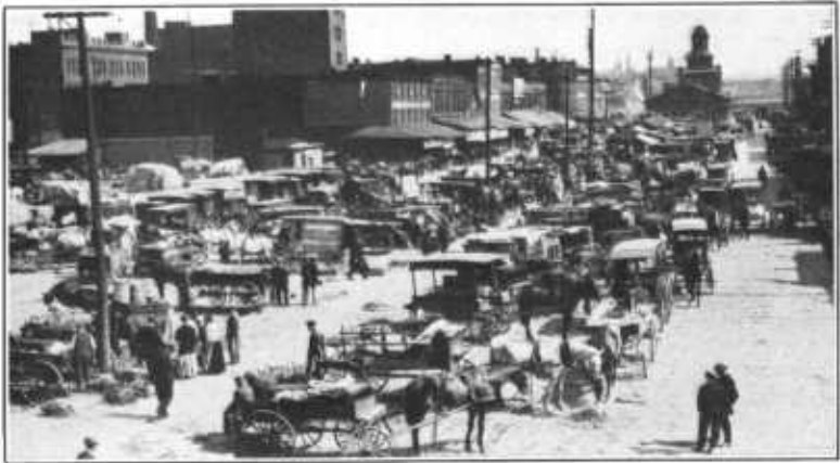
FIG. 1.—OPEN PART OF THE ELK STREET MARKET, BUFFALO, SHOWING INCLOSED BUILDING IN THE DISTANCE.
