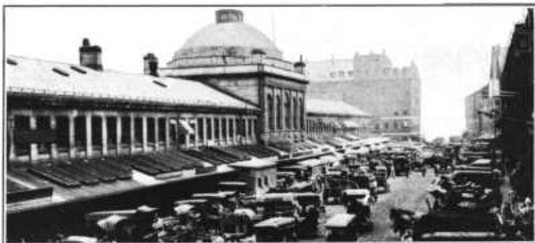
FIG. 3.—PORTION OF FANEUIL HALL MARKET IN BOSTON, SHOWING BUILDING FOR SALE OF MEATS, BUTTER, FISH, ETC., AND THE OPEN SPACE FOR PRODUCERS' WAGONS.
