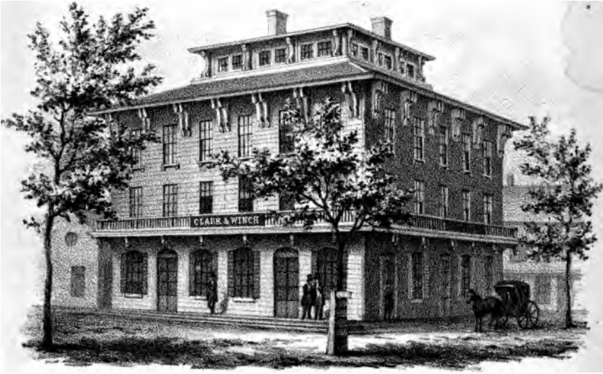
CLARK & WINCHRS BUILDING, CORNER MAIN & CENTRAL ST'S, NATICK.
