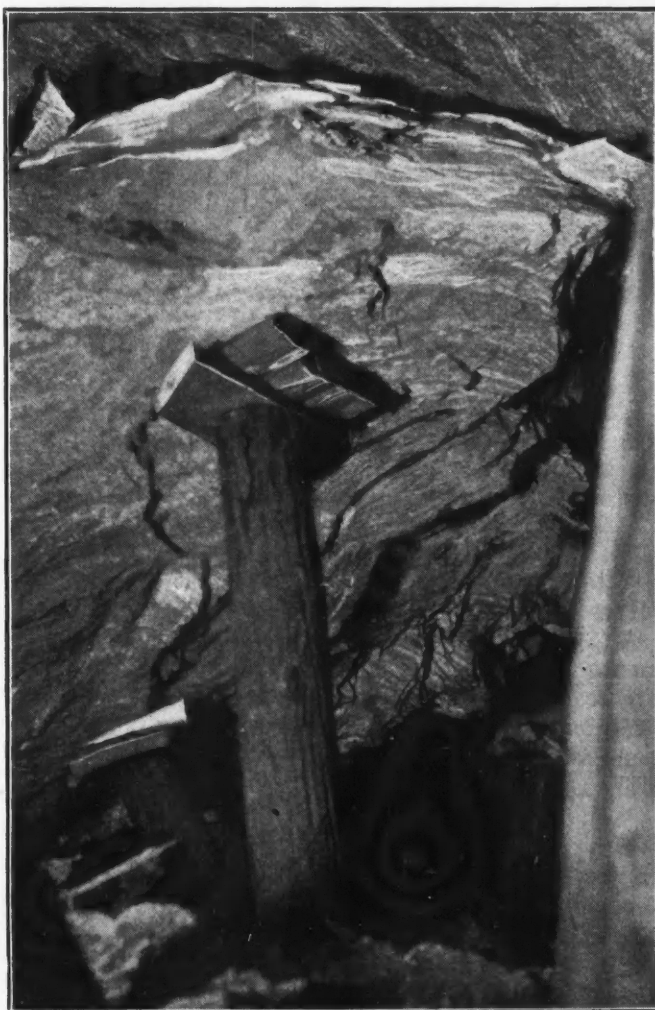
METHOD OF PROPPING BAD GROUND IN THE FRANKLIN MINE
