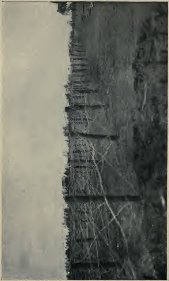
Antwerp was encircled by acres upon acres of barbed-wire entanglements. The wires were grounded and connected with the city lighting system.
