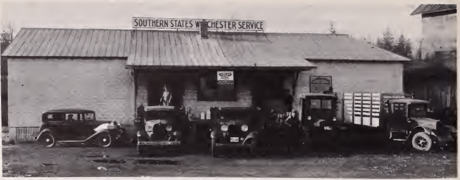
This picture was taken over 25 years ago at the Winchester, Va., service store of the Southern States Cooperative, Richmond, Va.
