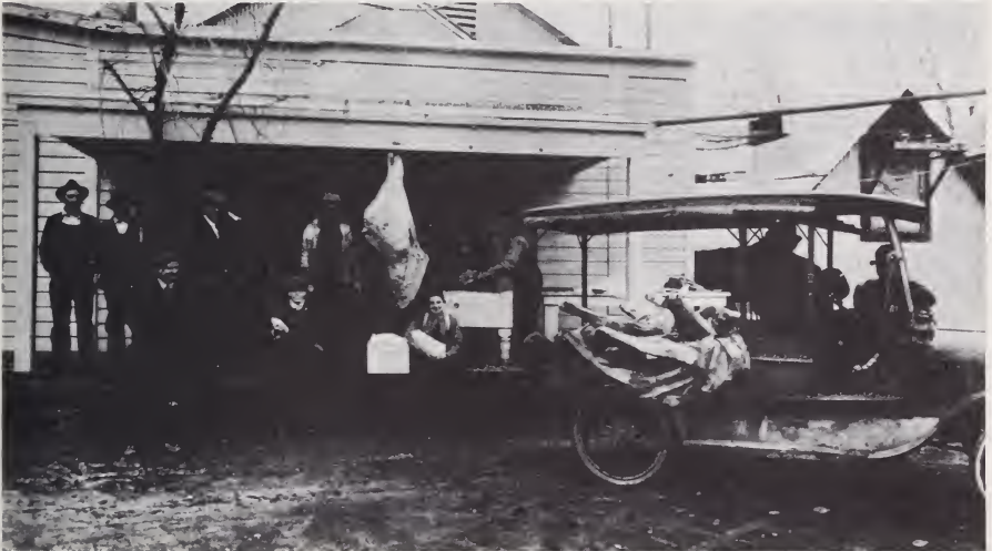
The Chico (Calif.) Ice and Cold Storage plant pictured here is believed to be the first frozen food locker plant in the United States. In front of the tree is the late Henry A. Eames, generally credited with using the frozen food storage idea in the early 1900's. In 1940, the Division established a Frozen Food Locker Section.
