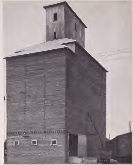
An early "crib" elevator in the Pacific Northwest. One of the earliest projects the Department of Agriculture undertook in the field of farmer cooperatives was to develop an accounting system for cooperative grain elevators.
