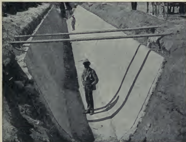
B. CEMENT LINING OF SANTA ANA CANAL, CALIFORNIA.
