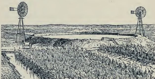
FIG. 87.— Windmill pumping into earth reservoir.
