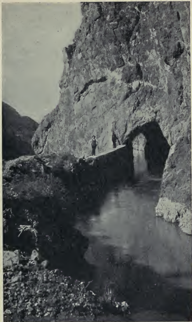
TUNNEL OF BEAR RIVER CANAL, UTAH.
