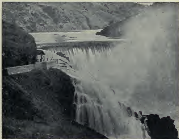
B. LAGRANGE DAM, WITH FLOOD PASSING OVER CREST AND SPILLWAYS.
