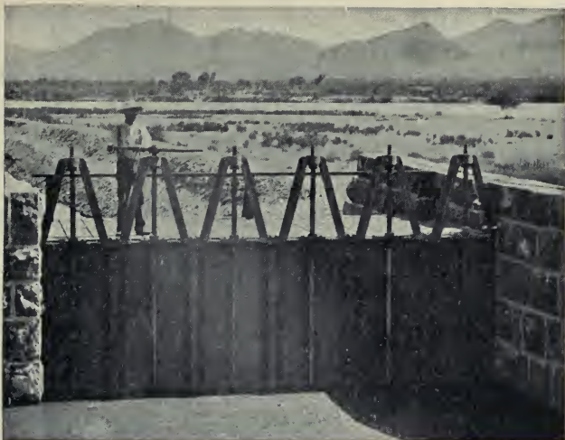
A. MASONRY HEAD-GATES OF CANAL.
