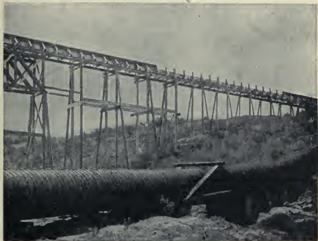
B. OLD FLUME AND REDWOOD PIPE REPLACING IT, REDLANDS CANAL, CALIFORNIA.
