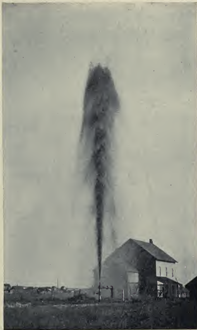
WELL AT WOONSOCKET, SOUTH DAKOTA, THROWING A 3-INCH STREAM TO A HEIGHT OF 97 FEET
