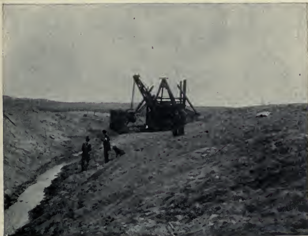
B. DREDGE CUTTING CANAL TO RECEIVE SEEPAGE WATER.
