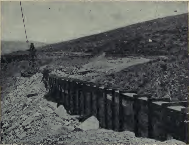
4. LOWER OTAY DAM, CALIFORNIA, SHOWING METHOD OF PROTECTING STEEL PLATES.
