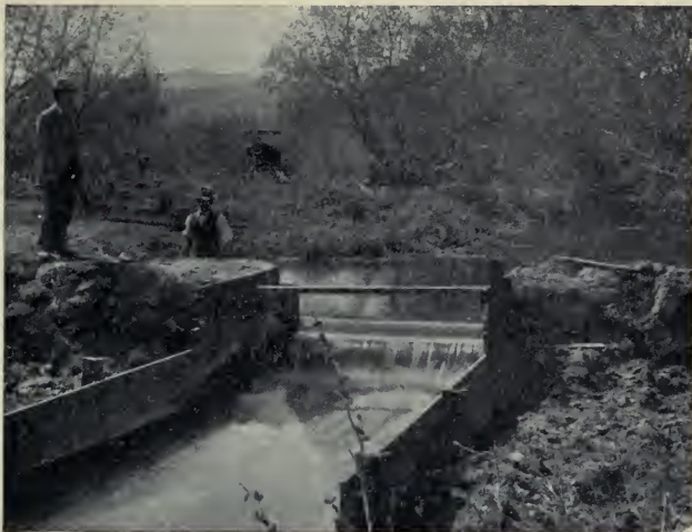
A. WEIR MEASUREMENTS OF LOS ANGELES RIVER IN SAN FERNANDO VALLEY, CALIFORNIA.
