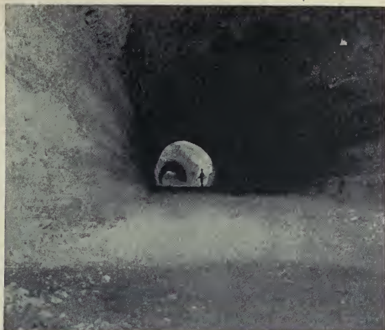
A. TUNNEL ON TURLOCK CANAL, CALIFORNIA.
