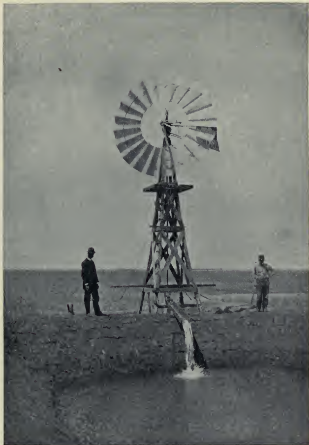
WINDMILL PUMPING INTO SOD-LINED RESERVOIR.
