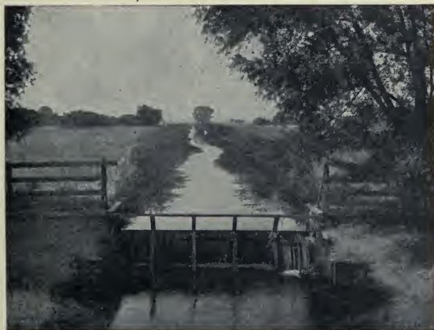
B. CHECK WEIR AND DROP.
