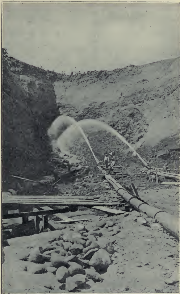
EXCAVATING DEEP CUT FOR CANAL BY HYDRAULIC PROCESS.
