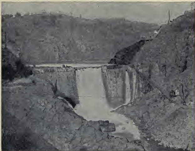
A. LAGRANGE DAM, NEARLY COMPLETED.
