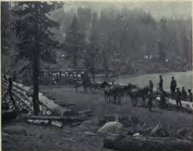
B. CONSTRUCTION OF TIMBER DAM AT BLUE LAKES, CALIFORNIA.
