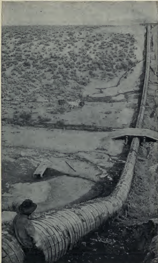
WOODEN PIPE LINE ON PHYLLIS CANAL, IDAHO.
