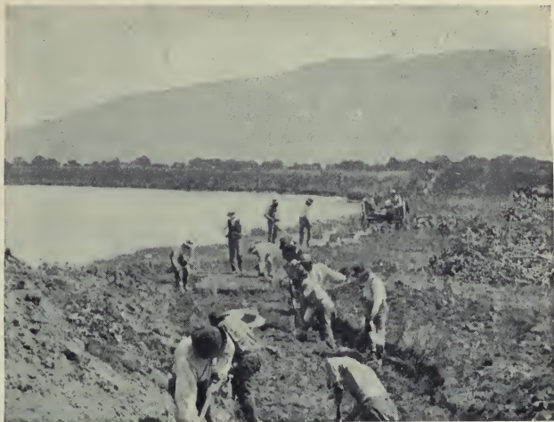
A. DIGGING A DITCH FROM A RIVER.
