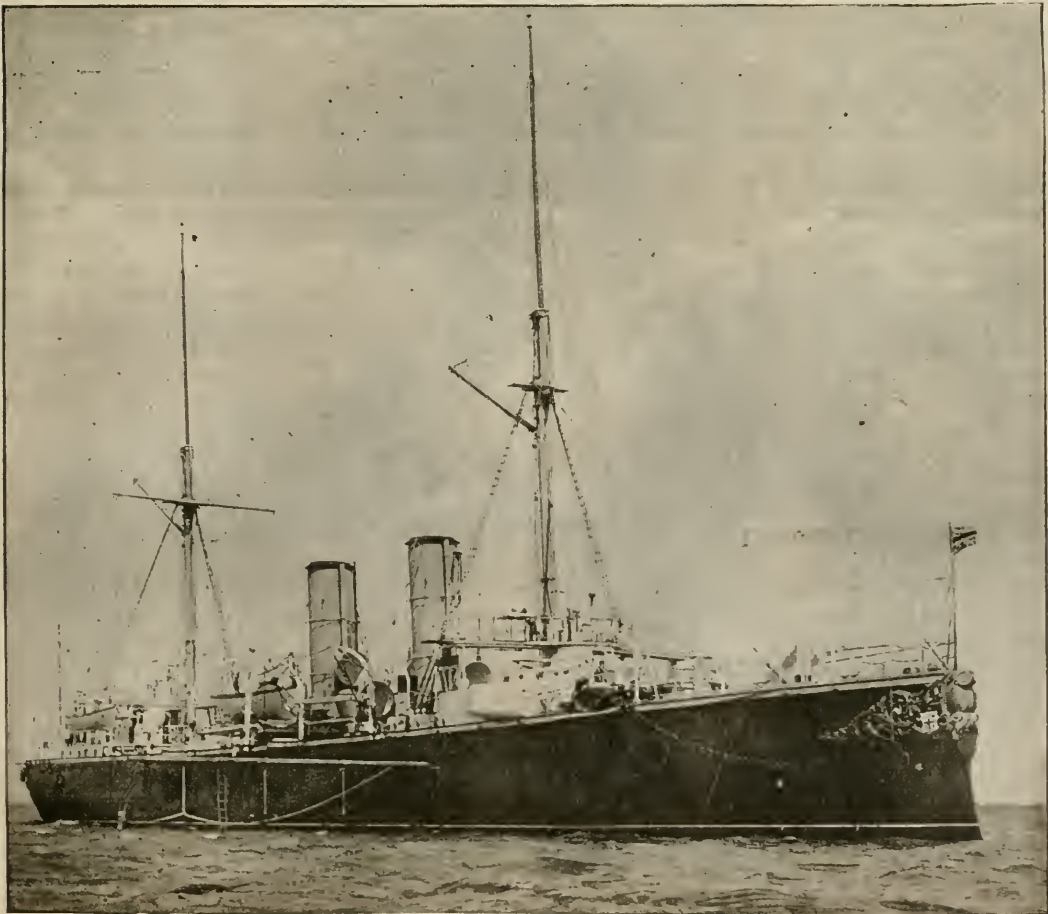
H.M.S. "KATOOMBA," 2nd CLASS PROTECTED CRUISER, ONE OF THE NEW AUSTRALIAN SQUADRON, 2,575 TONS, 7,500 HORSE-POWER.
