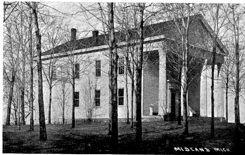
MIDLAND COUNTY COURT HOUSE, MIDLAND, MICH.
