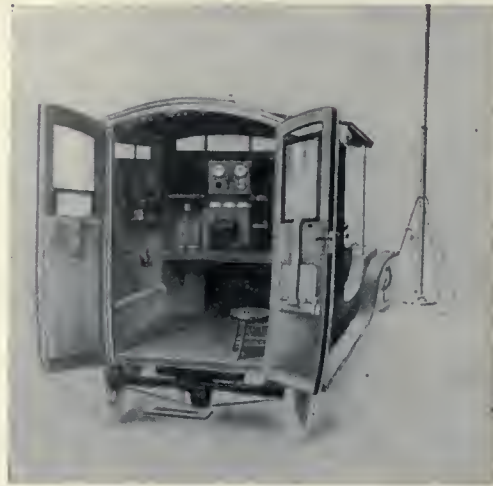
Fig. 12. A motor car wireless station.
