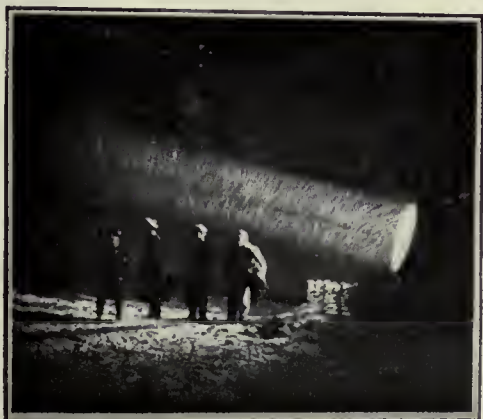
Powerful searchlight for illuminating hangars.
