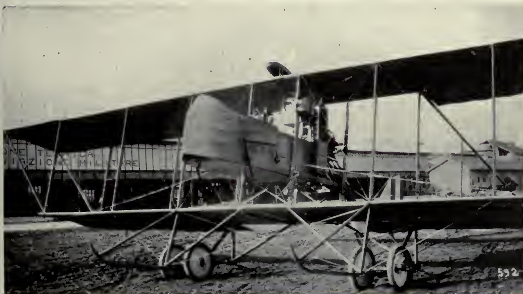
Aeroplane equipped with Sperry Automatic pilot.
