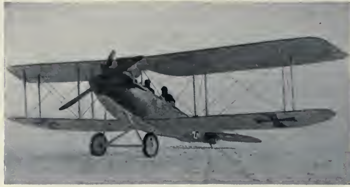
The German "Rumpler" biplane, two-seater, equipped with two guns.
