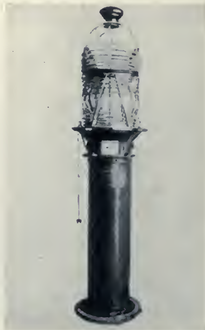
Aerial beacon with electric flashlight.
