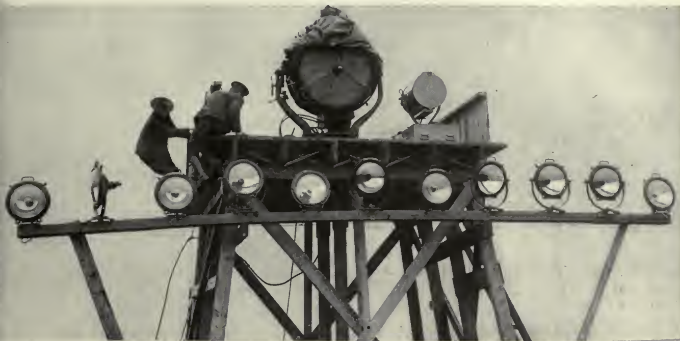
Lighting stand, serving the double purpose of guiding nocturnal flyers to a safe landing and detecting hostile aeroplanes.
