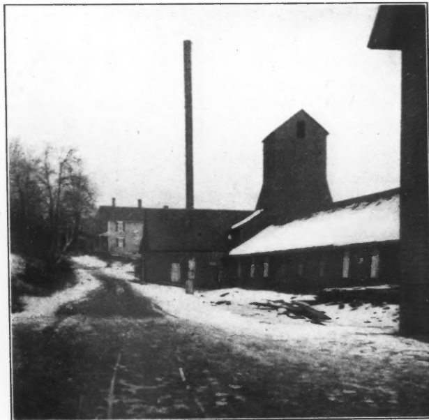
SHAFT HOUSE NO. 3 AND ORE SHED
