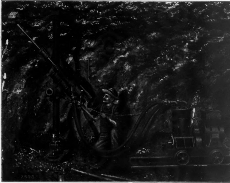
FIG. 1. VIEW OF ELECTRIC AIR DRILL
