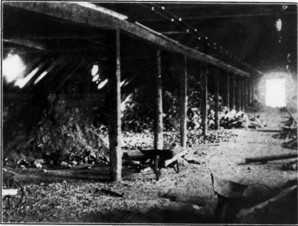
ORE SHED AT SHAFT NO. 1
