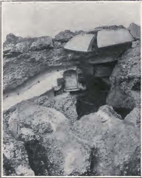
EFFECT OF GERMAN HEAVY SIEGE GUN FIRE ON LIÈGE ARMORED CUPOLAS
