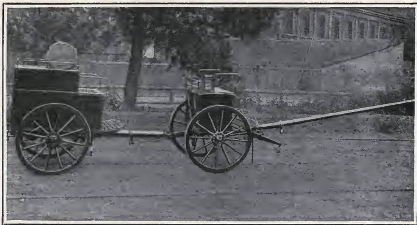
AUSTRIAN ARTILLERY CAR FITTED WITH ULTRA-VIOLET RAY STERILIZER
