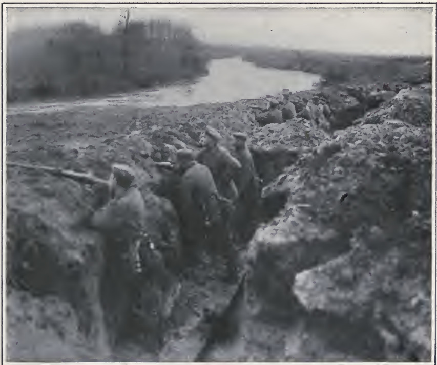
TRENCH, WITH TRAVERSES, BORDERING A STREAM
