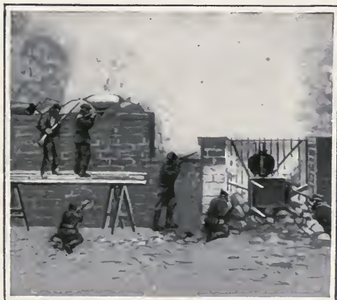
FIG. 26—LOOPHOLES MADE OF SANDBAGS. NOTE THE USE OF BARRICADES
