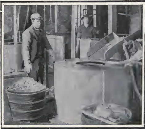
THE NITRATING HOUSE IS LIKE A GREAT, GLOOMY STEAM LAUNDRY—THE COTTON BEING DIGESTED IN CENTRIFUGAL WRINGERS LIKE THOSE IN WHICH CLOTHES ARE WASHED
