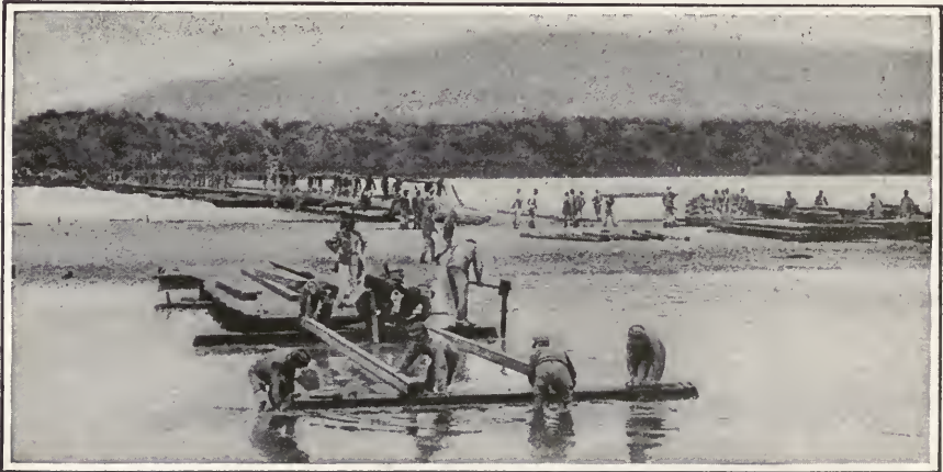
AUSTRIAN ARMY ENGINEERS AT WORK ON A PONTOON BRIDGE
