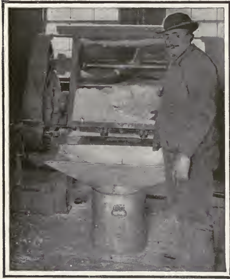
ONE OF THE MECHANICAL KNEADERS IN WHICH THE "PYRO" IS MIXED WITH ETHER-ALCOHOL SOLVENT, AND CONVERTED INTO "COLLOID," BEFORE PRESSING IT INTO SOLID CYLINDERS
