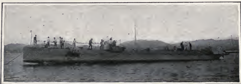
SUBMARINE "G. PULLINO." DISPLACEMENT, 400 TONS, SPEED, 13 SURFACE KNOTS, 9 SUBMERGED KNOTS. TORPEDO TUBES, 2
