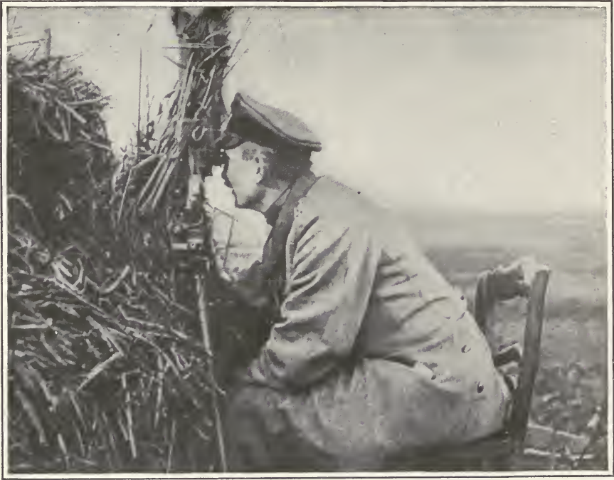
PERISCOPE FIELD-GLASSES CONCEALED BY A WISP OF STRAW
