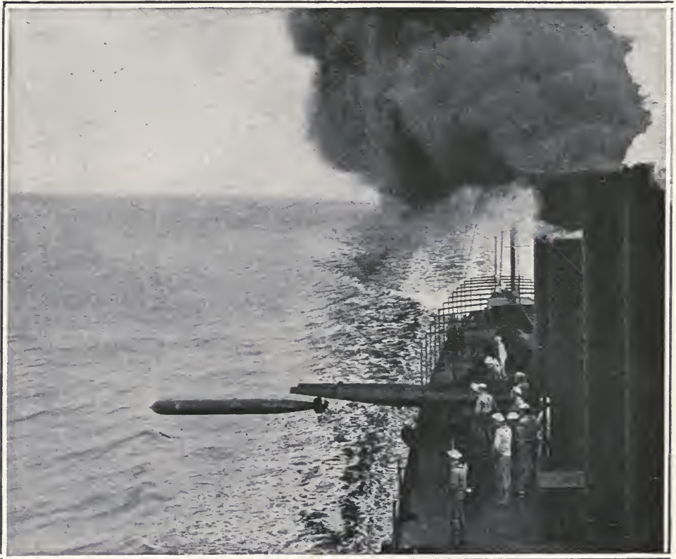
DISCHARGING A TORPEDO FROM A DESTROYER'S DECK TUBE
