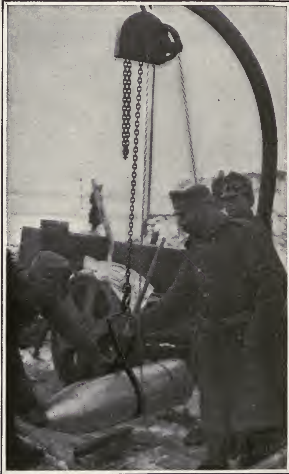
HOISTING THE 858-POUND SHELL INTO POSITION FOR LOADING
