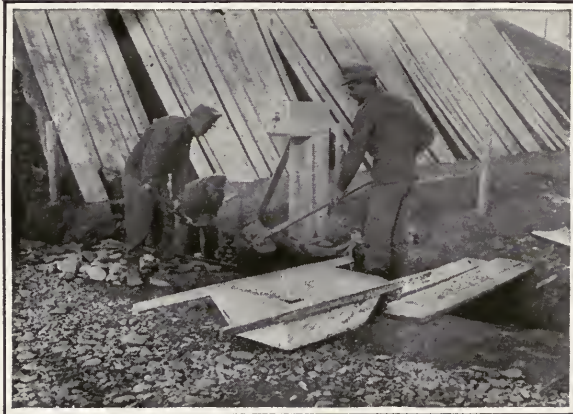
LIME DITCHES SURROUNDING BARRACKS IN WHICH CHOLERA PATIENTS ARE HOUSED
