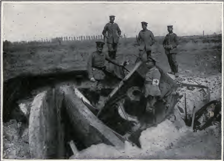
HIGH-EXPLOSIVE SHELLS BURSTING DEEP WITHIN THE EMPLACEMENT HAVE COMPLETELY INVERTED THIS GUN AND ITS TURRET
