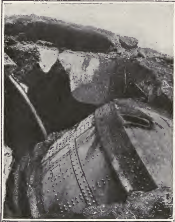
A LIÈGE CUPOLA THROWN FROM ITS MOUNTING BY GERMAN SIEGE GUNS
