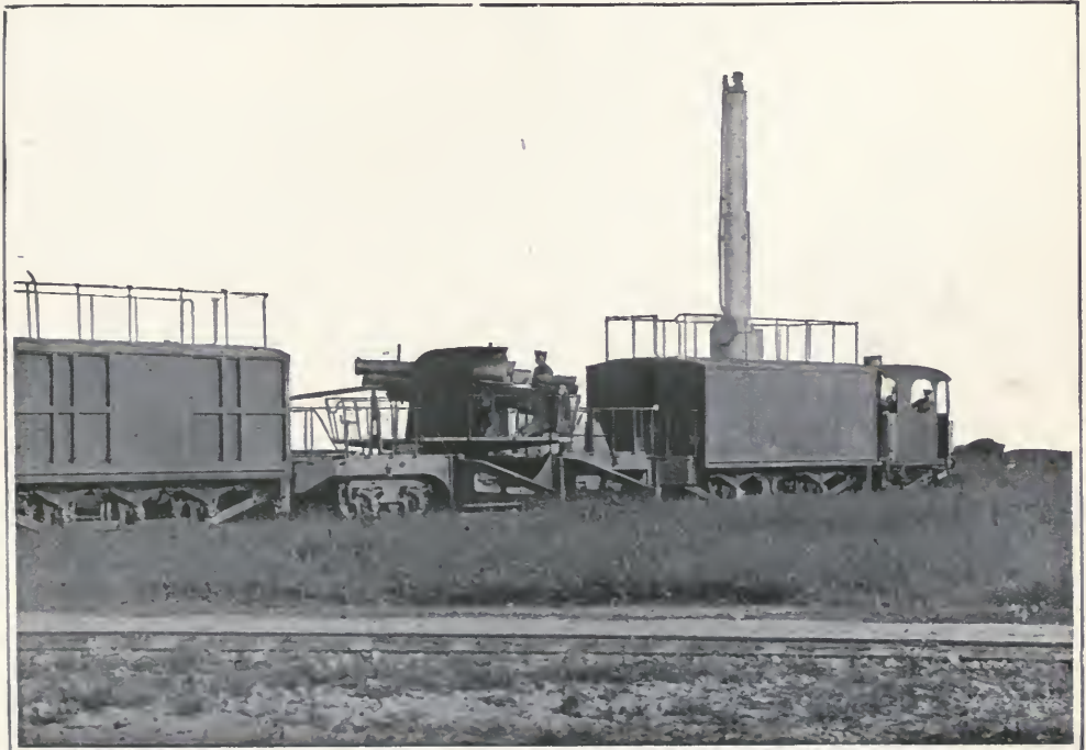
THE COMPLETE SCHNEIDER COAST DEFENSE TRAIN BATTERY. IN THE CENTER IS THE AMMUNITION CAR; ON EACH SIDE ARE THE TWO GUNS; AND TO THE RIGHT IS THE OBSERVATION CAR
