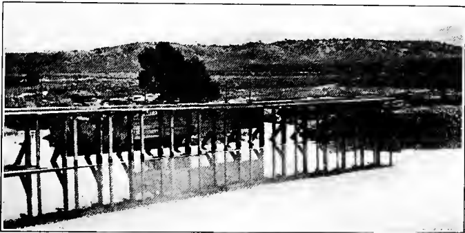
FIG. 19. — Reservoir for the storage of irrigation water.
