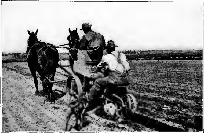
FIG. 62. — Potato planter at work: notched-wheel type.
