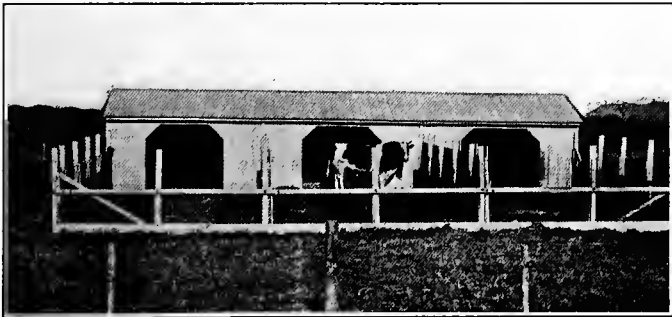
FIG. 96. — Cheap but effective shelter.
