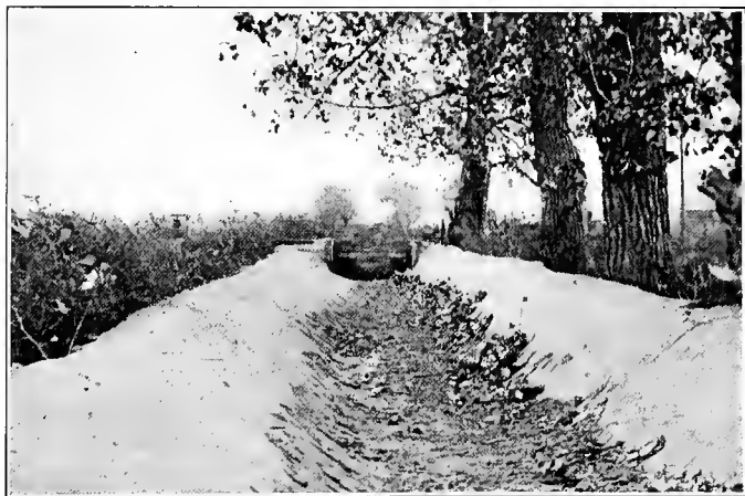
FIG. 21. — Cement lining prevents seepage.
