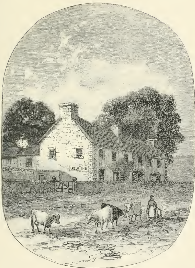
NEW INN, GRETA BRIDGE.
