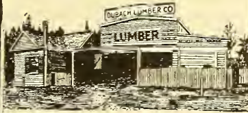
Covered with 15,000 ft. of Black Diamond Roofing.
