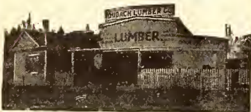
Covered with 15,000 ft. of Black Diamond Roofing.
