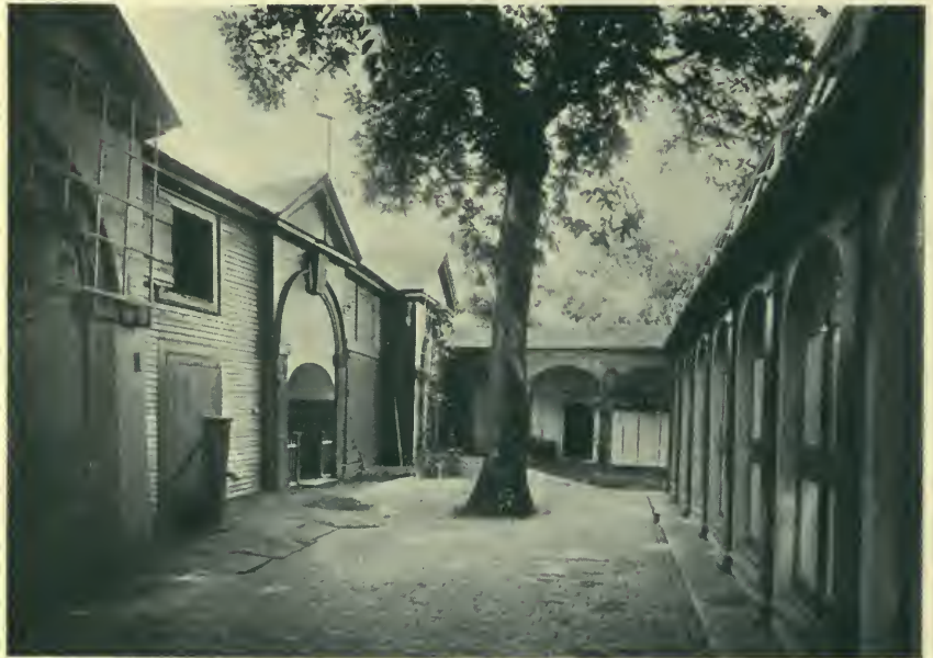
Courtyard. THE PIERCE-NICHOLS HOUSE, SALEM, MASSACHUSETTS.
