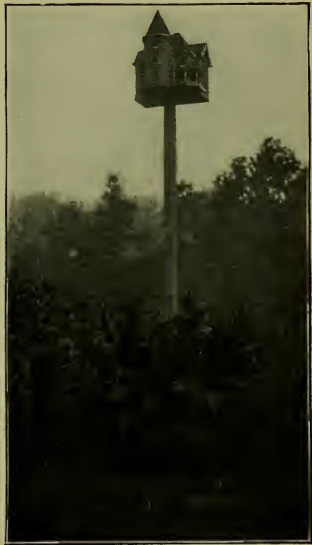
HOUSE NO. 2 IN POSITION
