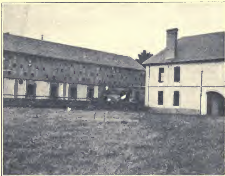
FIG. 2.—Camembert cheese factory at Lisieux, France. The square windows are seen in the second-floor rooms which are used in the first two weeks of ripening. (From Twenty-second Annual Report, Bureau of Animal Industry.)
