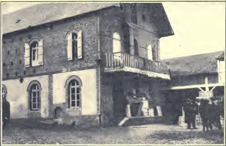
FIG. 6.—Another French factory, showing large windows, with blinds, in "sechoir" on second floor. (From Twenty-second Annual Report, Bureau of Animal Industry.)
