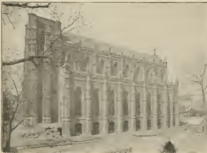
ST. FINBAR CATHEDRAL, BEING REBUILT.
