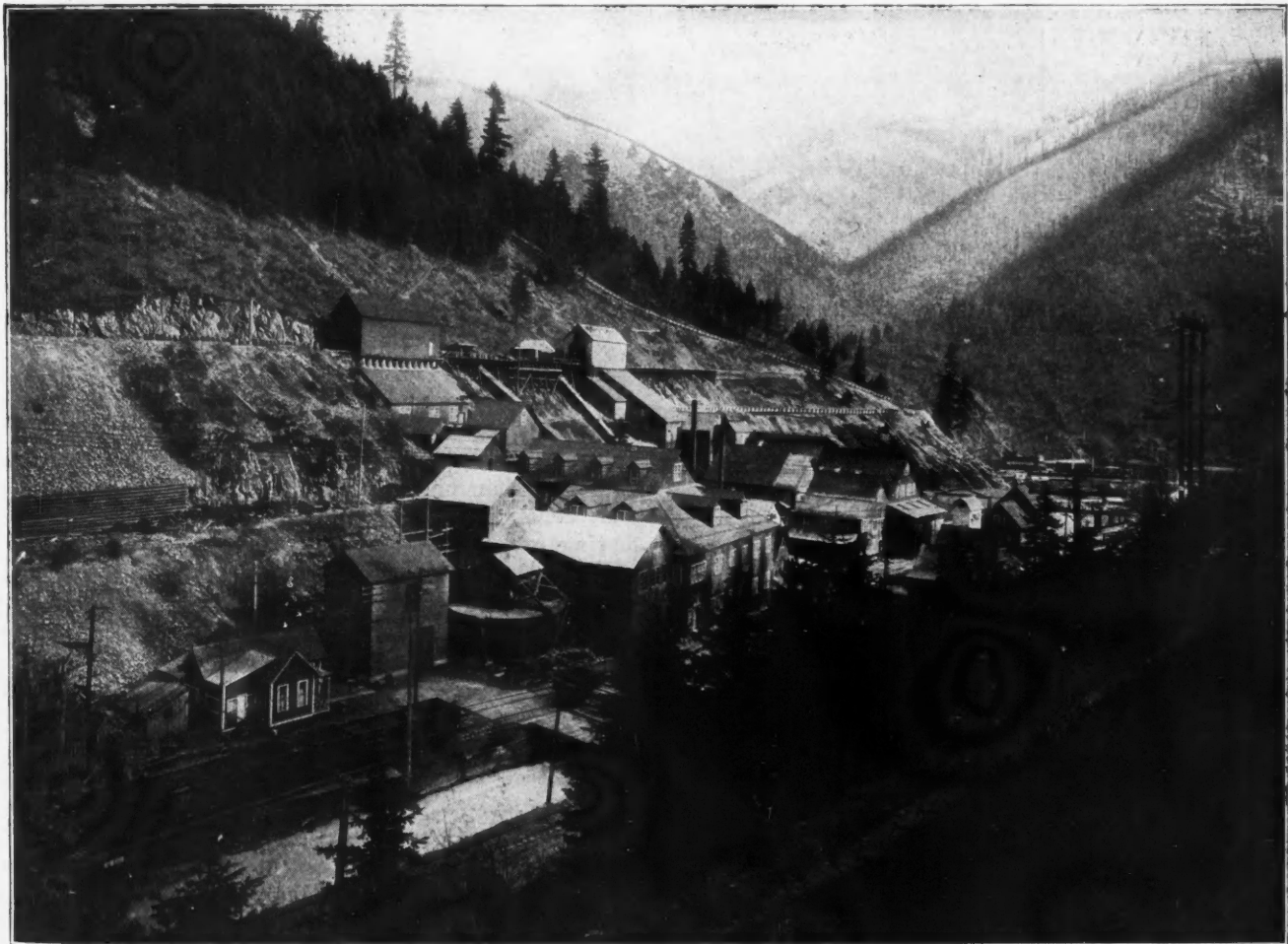
GREENHILL-CLEVELAND AND MORNING NO. 2 MILL, MACE, IDAHO
