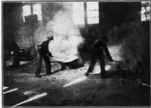
WORKING DROSS IN PERFORATED WHEELBARROWS
