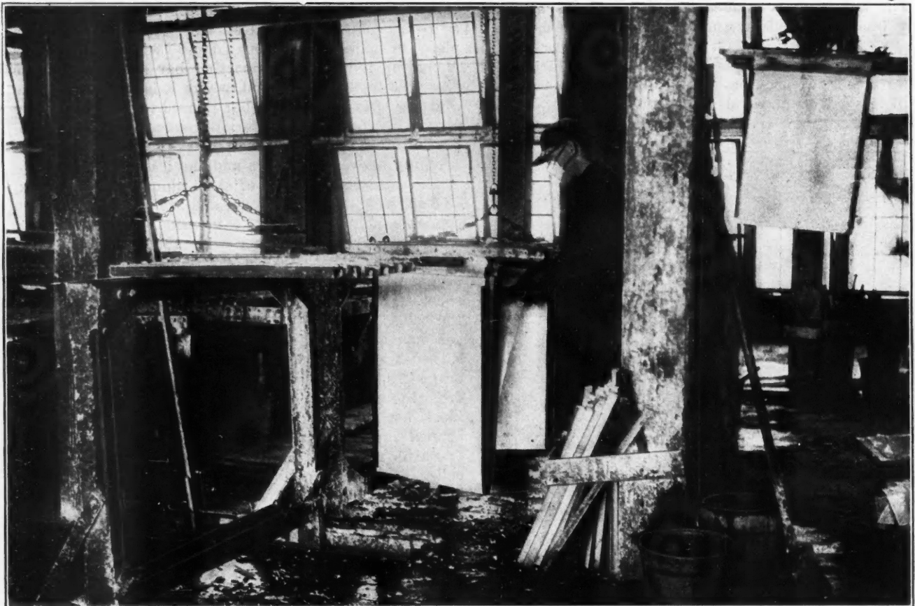
STRIPPING CATHODES IN THE ELECTROLYTIC ZINC PLANT
