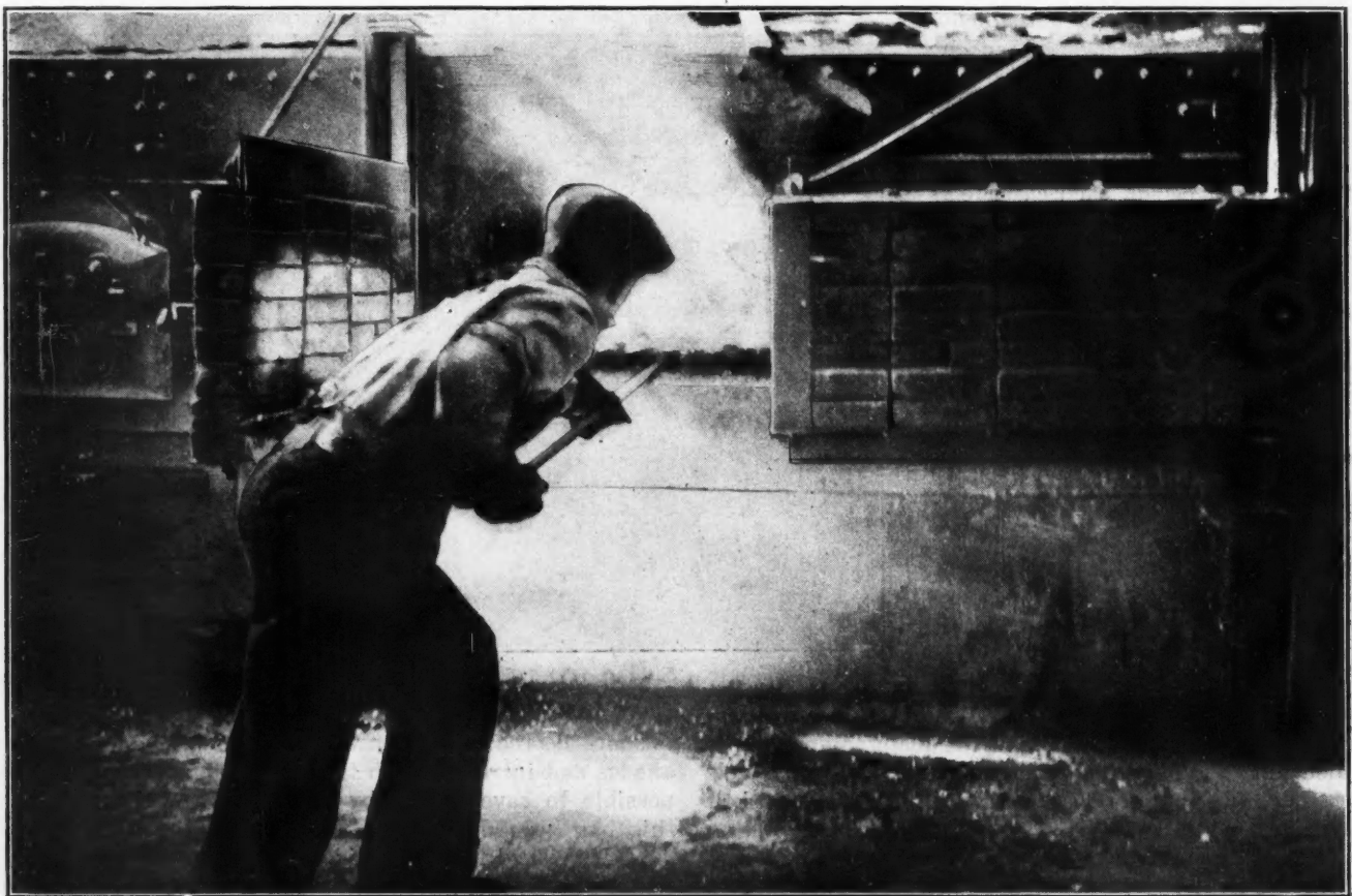
RABBLING THE DROSS IN A ZINC FURNACE
