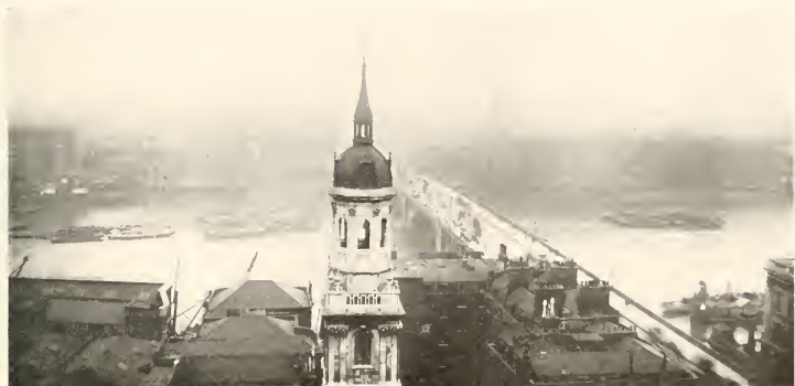
FIG. 206.—St Magnus from the Top of the Monument. (Looking across London Bridge.)
