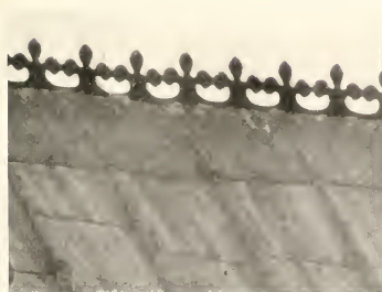
FIG. 188.—Lead Cresting, Exeter Cathedral.
