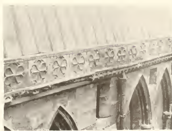
FIG. 189.—Parapet Gutter, Lincoln Cathedral.
