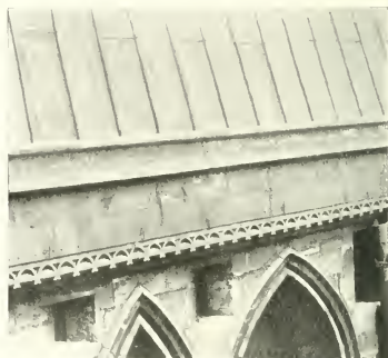
FIG. 191.—Leaded Parapet, Lincoln Cathedral.
