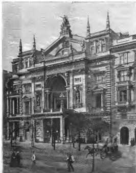
THE RING THEATRE, VIENNA, RECENTLY DESTROYED BY FIRE.—From a Photograph.—(See Page 574.)
