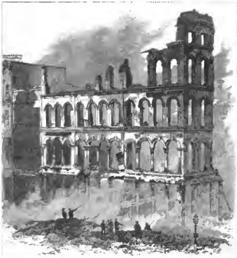
THE STRACON FIRE.—REMS OF THE WISTING OPERA-HOUSE.—From a Photograph at Nathan & Co's.
