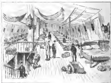
INTERIOR VIEW OF HOTEL BARGE.
