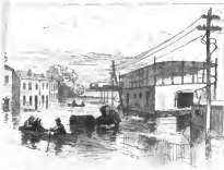
BOYER AVENUE, TEN FEET UNDER WATER.
