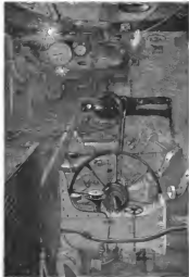
STEEL WORK—PREPARING TO LOAD.
