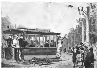
ELECTRIC RAILWAY AT BERLIN, GERMANY.
