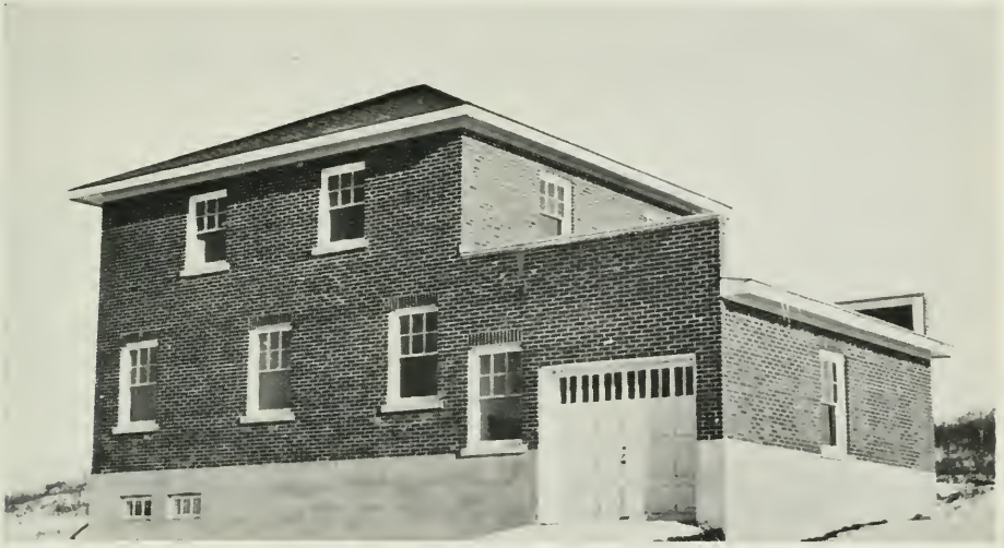
Sudbury Mine Rescue Station
