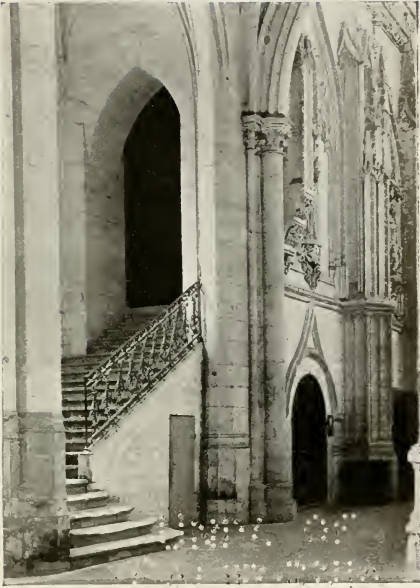
STAIRCASE IN CHOIR AISLE, ST. RIQUIER.
