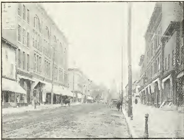
CHURCH STREET, Looking North.
