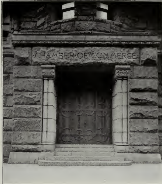
Main Entrance. To Corridors, Stairways and Elevators.
