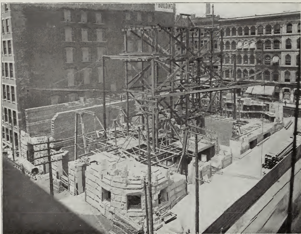
Early Stage of Construction, 1887, Showing Great Derricks.
