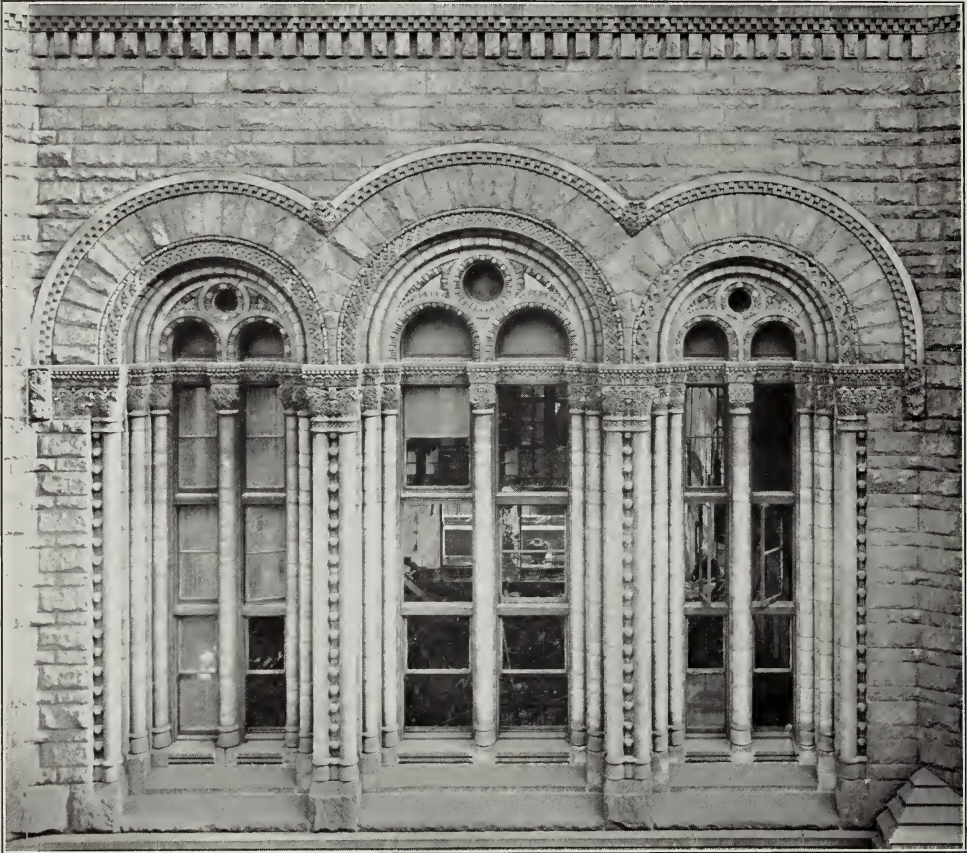
Fourth Street Window Arches, showing details of stone-carving. [Photo. by Longley, 1911]
