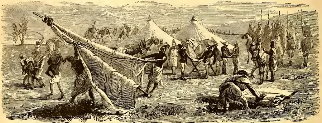
THE CARAVAN.—GETTING READY FOR AN EARLY START.
