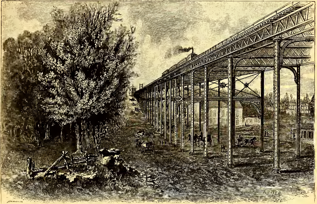
PORTION OF THE ROAD BEYOND CENTRAL PARK, ON POSTS FIFTY-SEVEN FEET HIGH.
