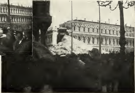
NO. 2. SAME VIEW AS NO. 1. AFTER THE FALL OF THE TOWER.
