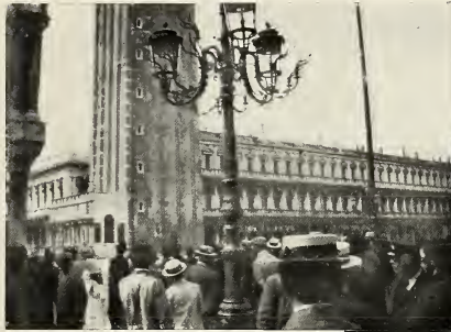
NO. 1. THE TOWER A FEW MINUTES BEFORE IT FELL
