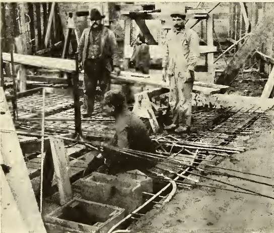
FIG. 3. SHOWING HOW THE FLOORS ARE REINFORCED BY IRON RODS BEFORE THE CONCRETE IS POURED OVER THEM.
