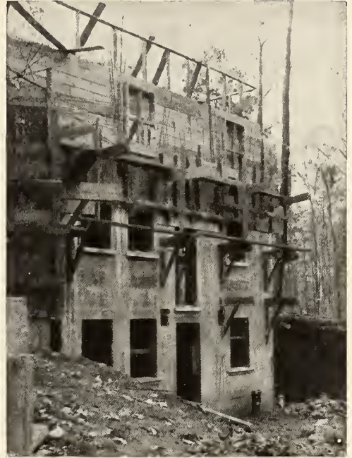
FIG. 2. THE WOODEN MOLDS IN PLACE FOR CASTING THE THIRD STORY WALLS.
