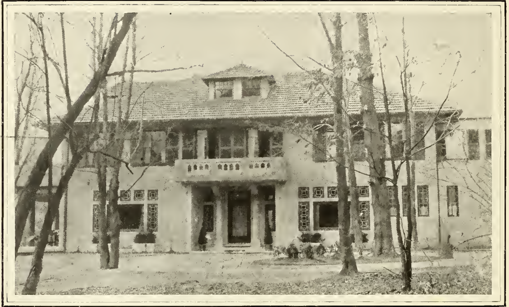
FIG. 4. A CONCRETE HOUSE, COMPLETED.
