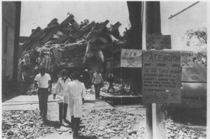
Sign cautions workers to "touch cadavers with gloves only."
