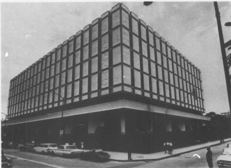
The embassy. (State Department photo.)
