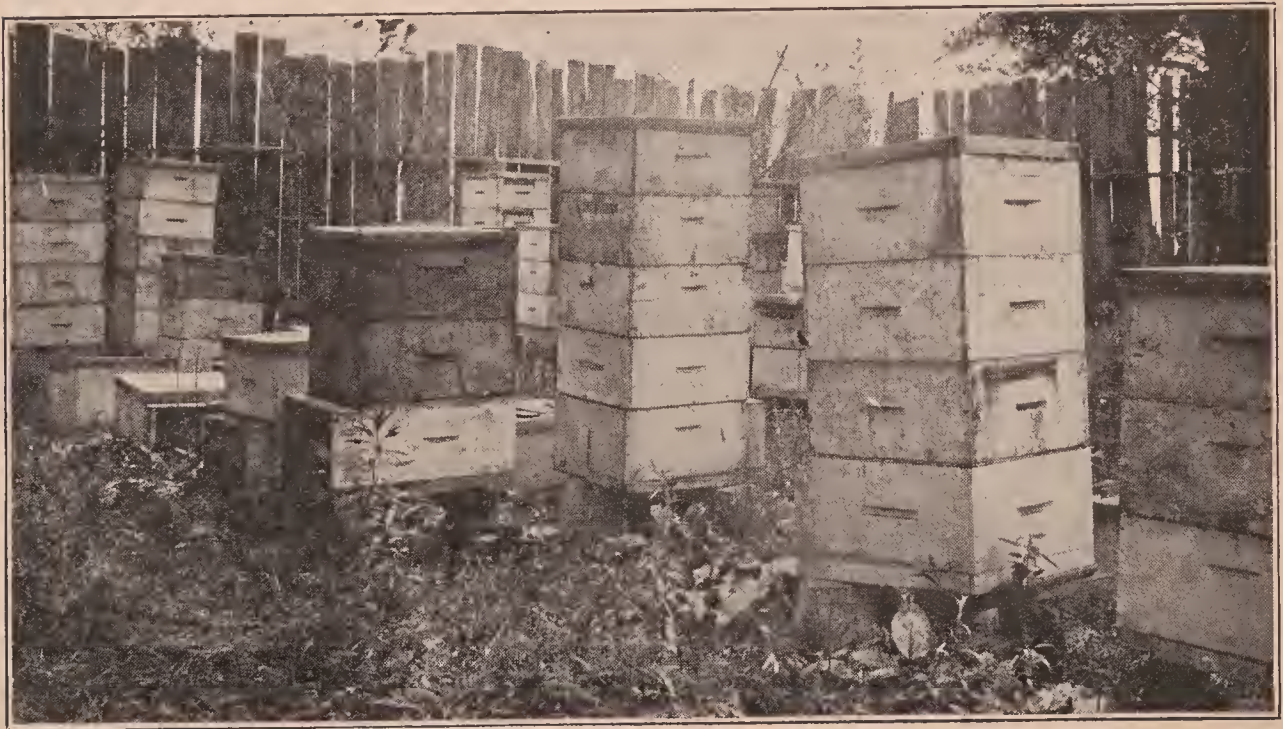
Fig. 2.—Twelve-foot fence windbreak used by R. F. Holtermann. The boards are nailed vertically on to horizontal cross pieces nailed or bolted on to the posts. This construction can be made up in panels so that the fence can be moved in sections if necessary.
