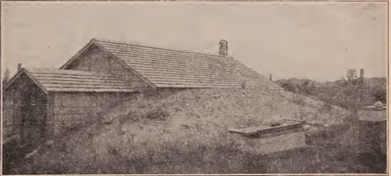
Fig. 3.—This cellar belongs to L. C. Gordon, of Bellaire, Mich. According to David Running's idea the roof should have extended over the side embankment. But these embankments are made up of sand that dries out very quickly; and in spite of the fact that it is not covered, it makes a good insulator. Mr. Gordon once told the author that in this 12 x 20-foot bee-cellar the preceding winter he wintered 151 colonies without the loss of a colony. This cellar has the ventilation recommended by Mr. Running.
