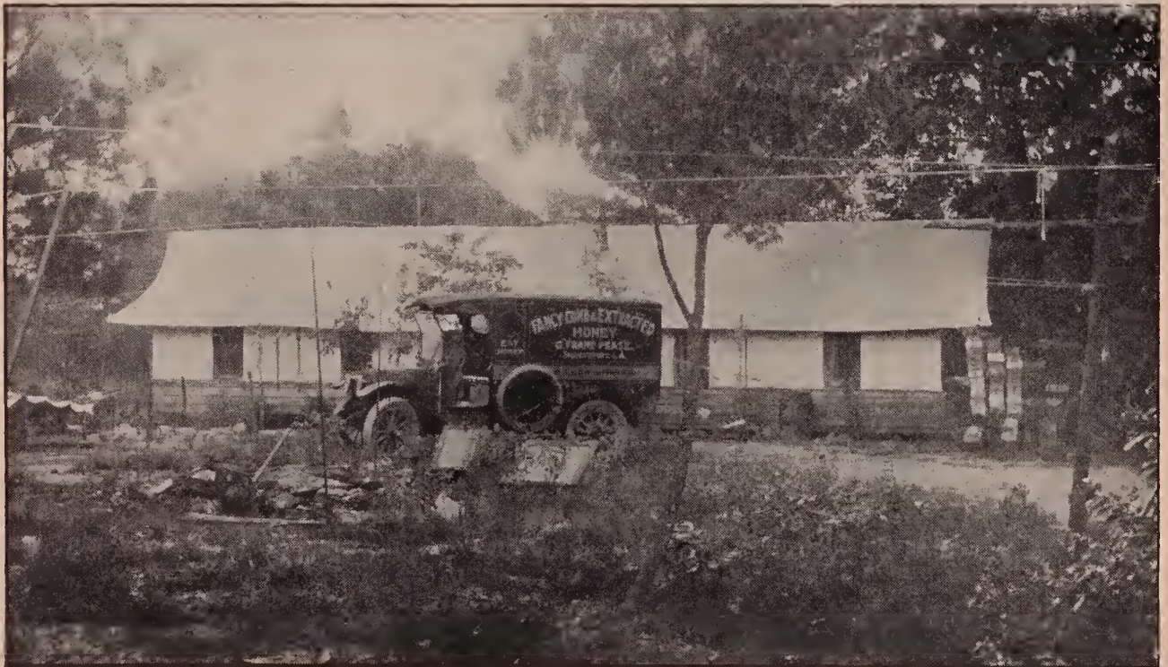
An inexpensive and quickly constructed building that answers every requirement. Walls and floor of wood, roof of canvas. A good canvas roof gives a better light inside and is cooler than a solid roof.
