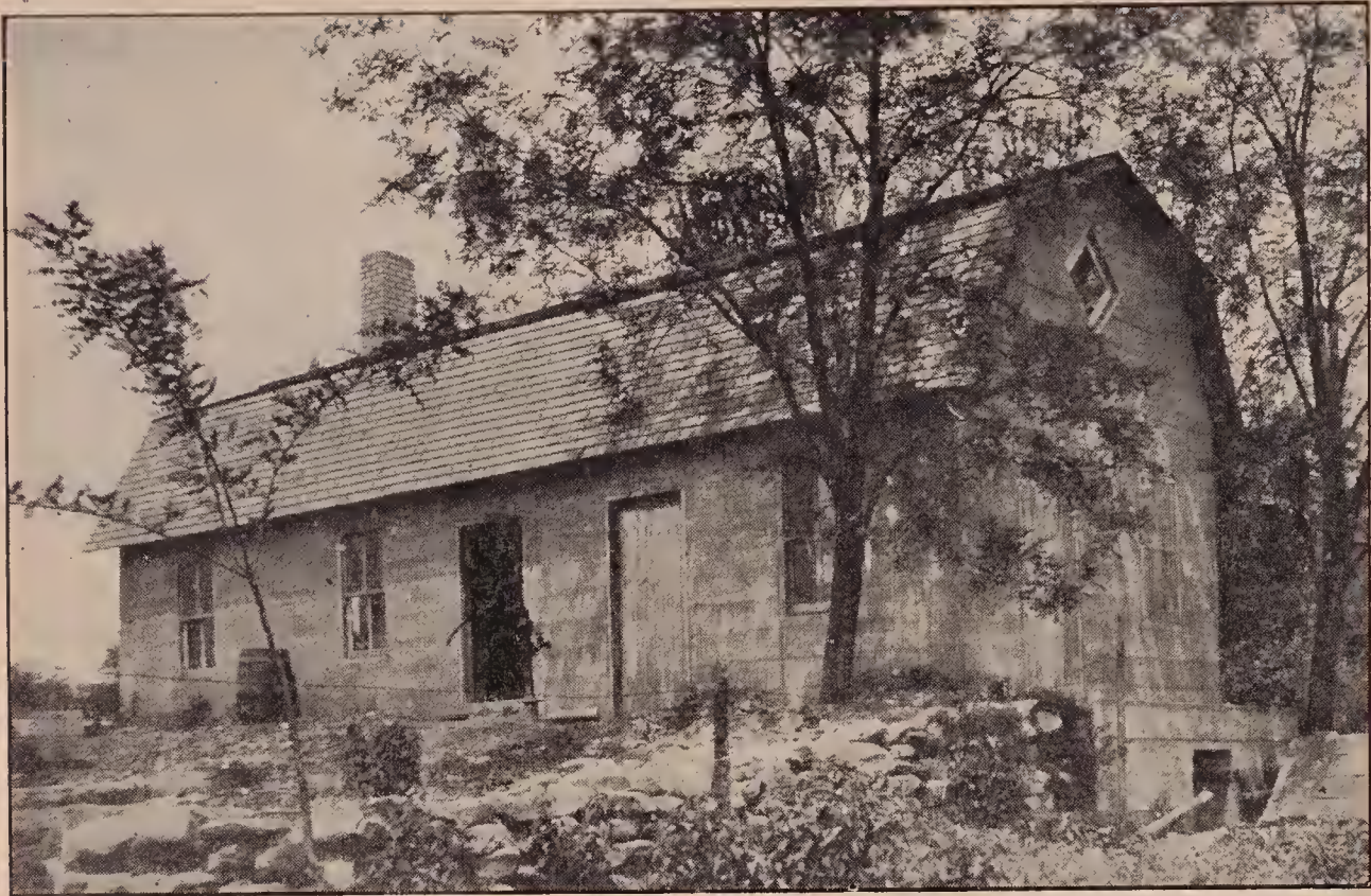
David Running's 16 x 40-foot concrete building. There are two different floors besides the cellar where the bees are wintered. The cellar has a capacity for nearly 350 colonies. Where gravel is cheap, concrete is cheaper than lumber in the long run.
