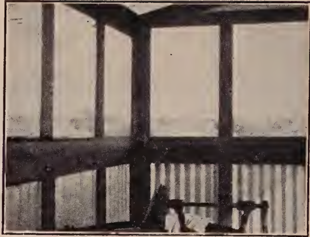
Interior of building. It is held together by barn-door hasps and wooden pegs on the inside of the corners. The windows are wooden frames with wire screen.
