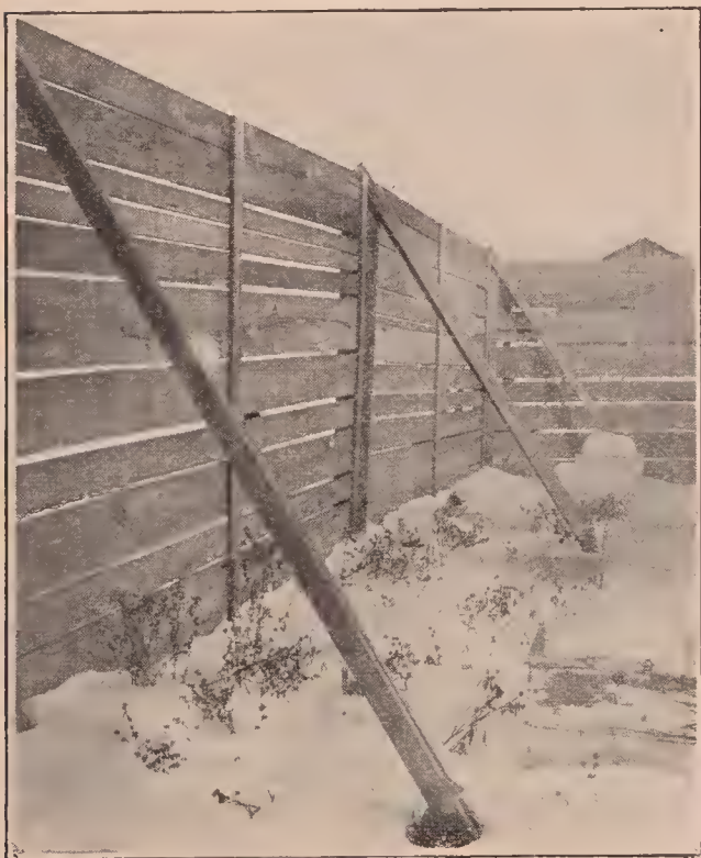
Fig. 8—Showing details of construction of an artificial windbreak. It will be seen that the windbreak is made up of panels, the boards of which are placed about an inch apart, each panel being held in place by means of braces on the outside and inside. The arrangement makes it possible to move the windbreak as well as the apiary itself. The panel is separated, the braces loosened, when the whole is laid on a truck.
