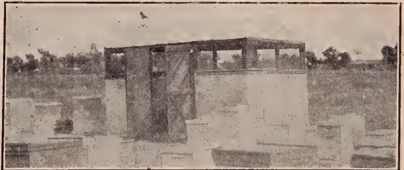
Dismantlable extracting-house of Frank McNay, Pasadena. This is made of four large panels or frames covered with cloth and mosquito netting. It is held together at the corners by means of large metal hinges. When it is desired to move, the bolts to the hinges are withdrawn, when the two sides of the hinges come apart, releasing the frames, when they are loaded one by one on to a truck. This building is very cheap and serviceable.
