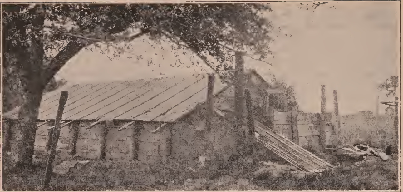
Fig. 2.—This is a bee-cellar belonging to Leonard Griggs, Flint, Mich. It is a type of an above-ground cellar embodying the ideas of David Running. The cellar proper extends into the ground about 3 feet. Then there is a three-foot embankment about 3 feet wide around the upper part of the cellar. The ceiling is covered with about 3 feet of sawdust. To keep the side embankments dry and frost-proof the roof extends entirely over the cellar, and the embankment, except in front; and Mr. Griggs thought it would be a good idea to cover this also. He has been uniformly successful in wintering bees in this cellar.
