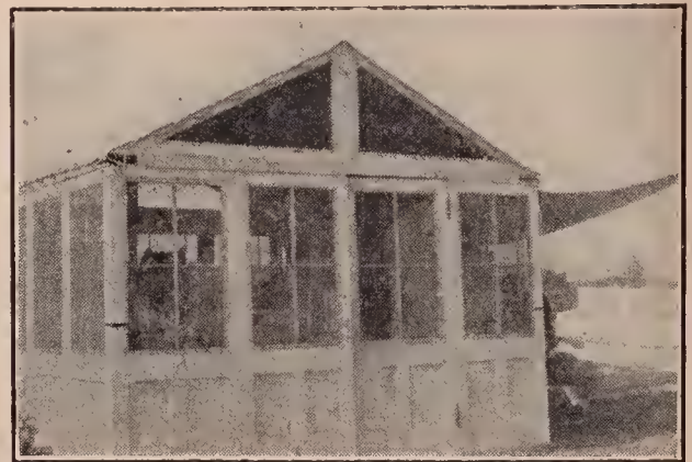
Portable extracting-house of A. F. Tice, Los Angeles, also shown in another cut. This structure is made up of door panels held together by clamps and bolts. The fact that Mr. Tice is a carpenter and builder explains why it is so neat and well designed. It is one of the best portable dismountable extracting-houses in California.
