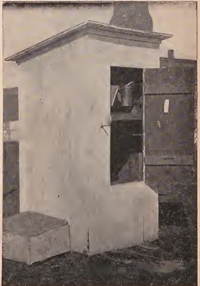
Fig. 3—A tool house for smokers, tools, veils, and fuel. The fuel is kept in the lower part under the shelf.
