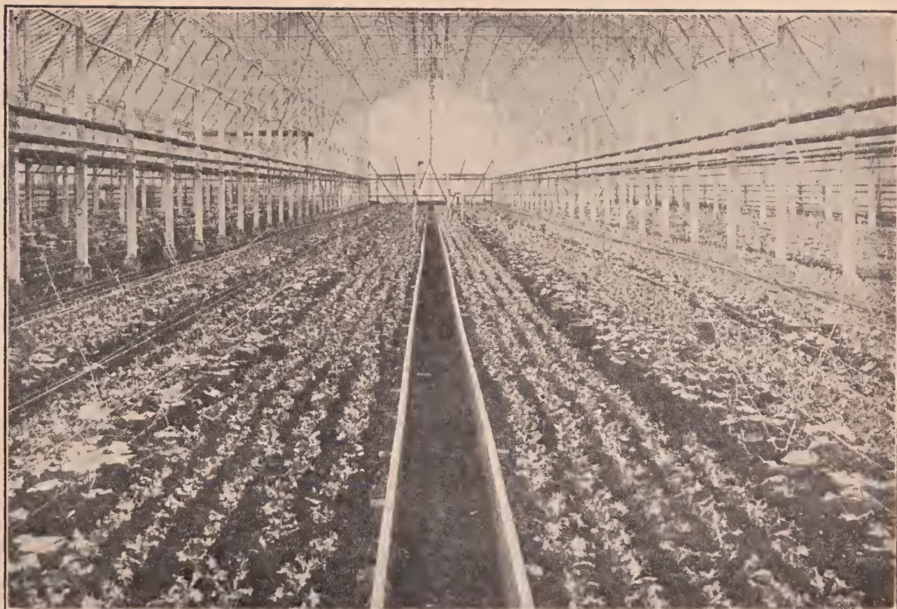
One-half of the great glass building at Ashtabula, Ohio. Cucumbers are replacing the lettuce and there are thousands of the golden yellow blossoms yielding to the bees their pollen and nectar. Many of the blossoms are visited by two or three bees in five minutes. The results show that the cucumbers are not only more perfect in shape but that the crop is much larger.
