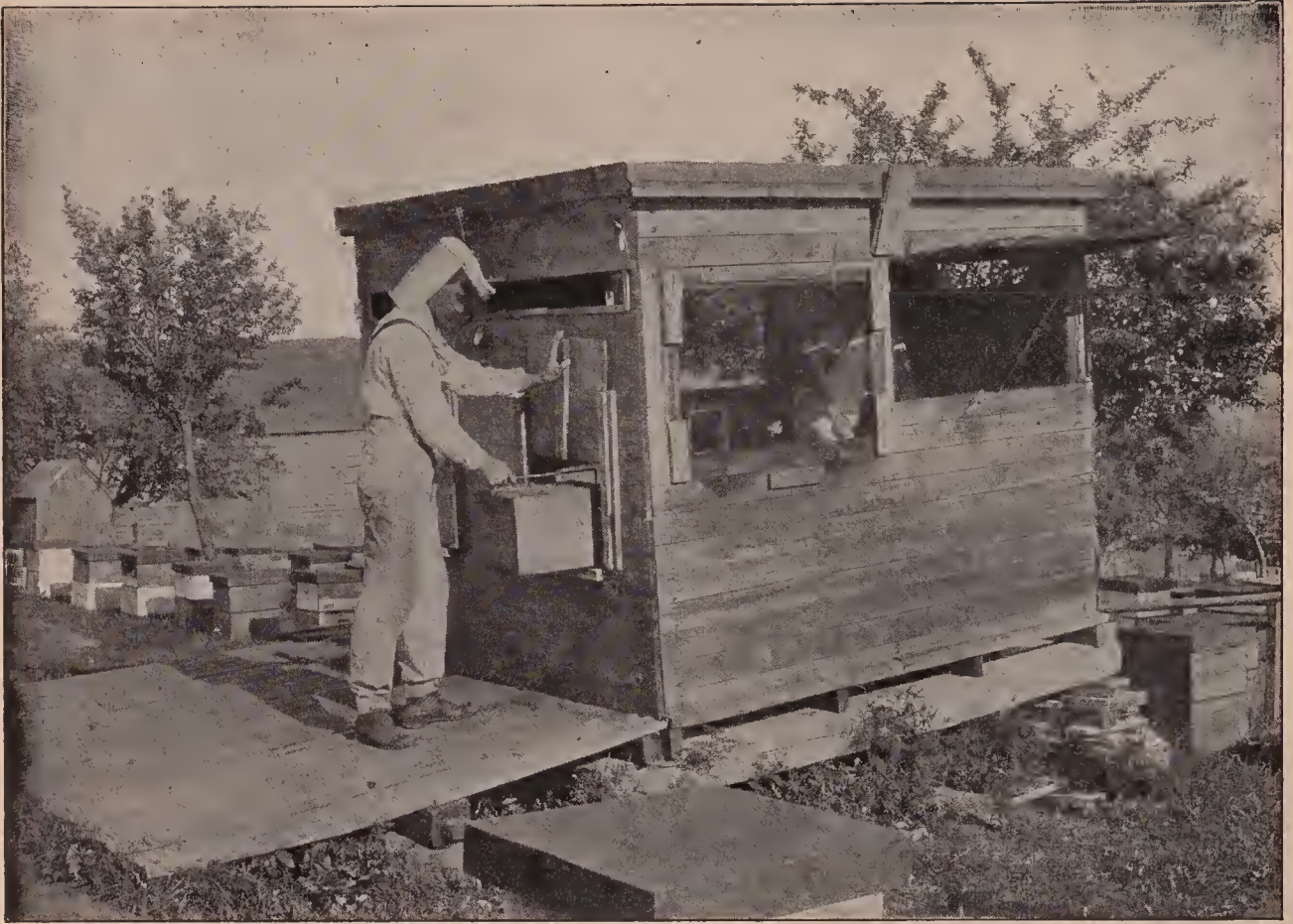
A small inexpensive extracting-room as formerly used by E. W. Alexander of Delanson, N. Y. There are two openings in the end of the building that close with sliding doors. The full combs are put in thru one door, and the empty ones taken out the other one. A pipe conveys the honey from the extractor to a tank in another building down the hill.
