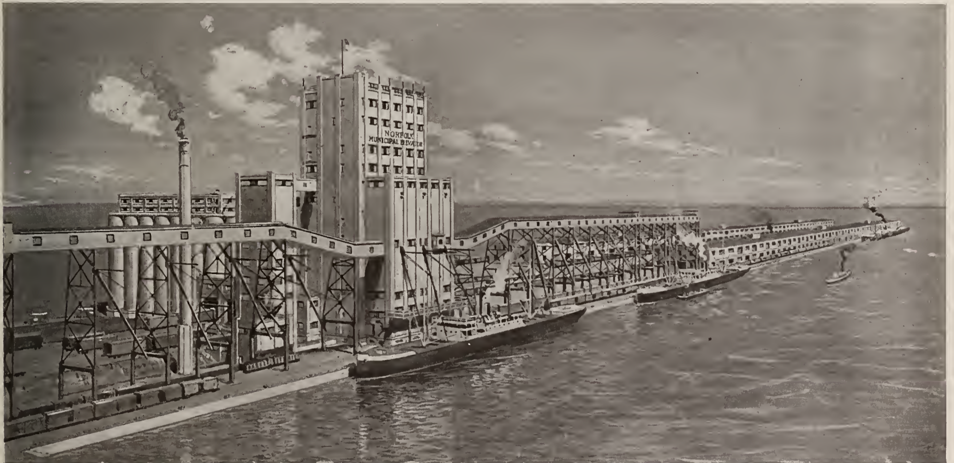
THE NEW MUNICIPAL ELEVATOR AT NORFOLK, VA., NOW UNDER CONSTRUCTION
