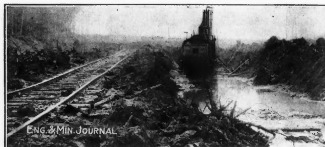
TAKING THE FIRST CUT IN STRIPPING BOGGY GROUND
