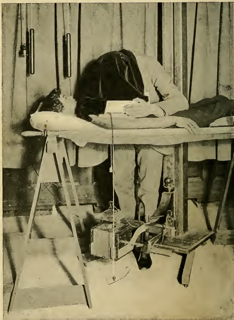
FIG. 59. This cut shows the method of examining the whole thorax with a large open screen, 30 by 35 centimetres, placed in a shallow box, the side of which is shown under the hand, the dark cloth being drawn aside for the purpose. The method here shown is the best for comparing one side of the thorax with the other. The observer is standing on the left side of the patient, in order that the latter may be visible. The observer should stand on the right side and have one hand on one of the long handles seen above the patient's head, as by this means the amount of light, which should be varied as the examination proceeds, is controlled.
