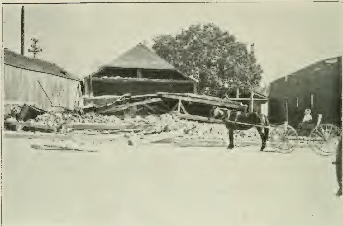
FIG. 13. BUILDINGS IN THE BUSINESS DISTRICT OF SAN JACINTO, CALIFORNIA, WRECKED IN AN EARTHQUAKE ON APRIL 21, 1918. (Photograph by Homer Hamlin.)
