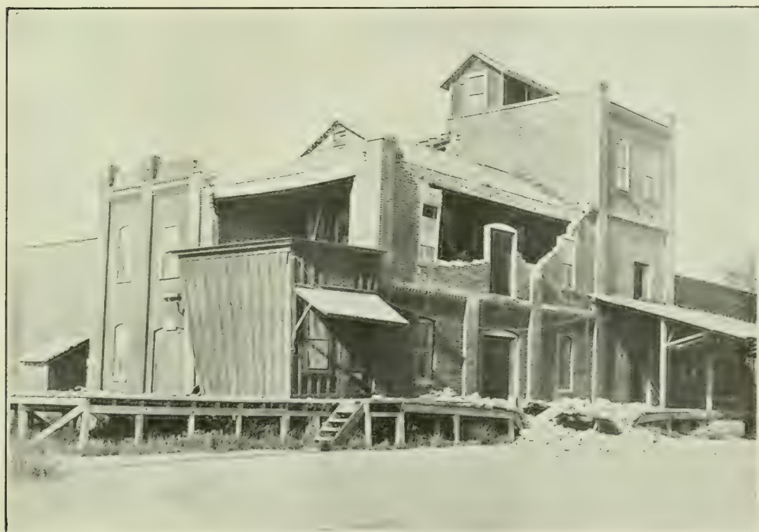
FIG. 4. A VIEW OF A FLOUR MILL AT HEMET, CALIFORNIA, SHORTLY AFTER THE EARTHQUAKE OF APRIL 21, 1918. Brick and adobe buildings can not withstand severe earthquakes, whereas reinforced concrete and steel frame buildings will stand through the strongest shocks. (Photograph by S. D. Townley.)
