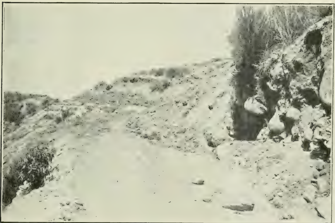
FIG. 12. THE ROAD BETWEEN HEMET AND IDYLVILD, CALIFORNIA, BLOCKED BY LANDSLIDES IN THE EARTHQUAKE OF APRIL 21, 1918 (Photograph by Homer Hamlin.)
