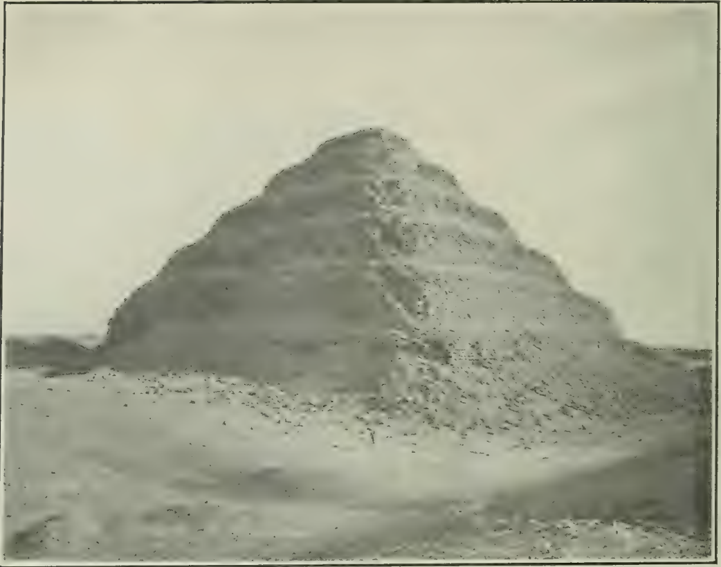
FIG. 66. TERRACED TOMB STRUCTURE OF PHARAOH ZOSER AT SAKKARA, EGYPT. The oldest known superstructure of stone,—built by the architect Imhotep (30th century B.C.).
