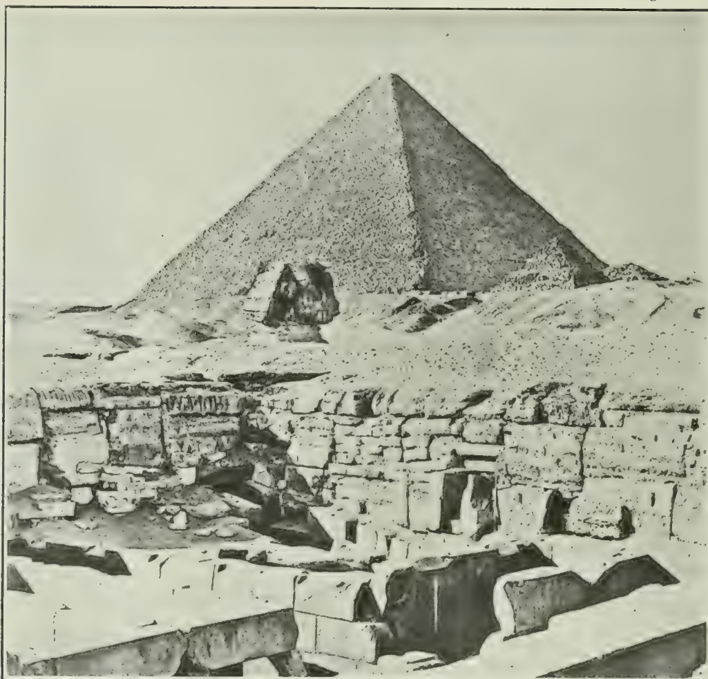
FIG. 79. INCIPIENT CLERESTORY IN THE HALL OF THE VALLEY TEMPLE OF KHAFRE AT GIZEH BUILT IN THE 29TH CENTURY B.C. The narrow light-chutes occupying the difference in level between a higher roof over the nave and a lower roof beside it are the lineal ancestors of the clerestory windows of European architecture. The oblique light which they admit is seen in Fig. 80.
