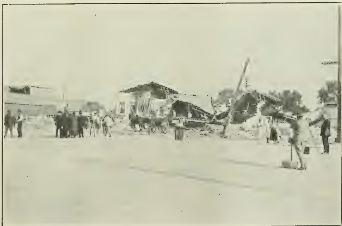
FIG. 14. STORE BUILDINGS IN THE HEART OF SAN JACINTO, CALIFORNIA, WRECKED BY AN EARTHQUAKE ON APRIL 21, 1918. Because of the fortunate time of occurrence, at 2:32 o'clock on a Sunday afternoon, the business district was largely deserted, and no lives were lost. (Photograph by Homer Hamlin.)
