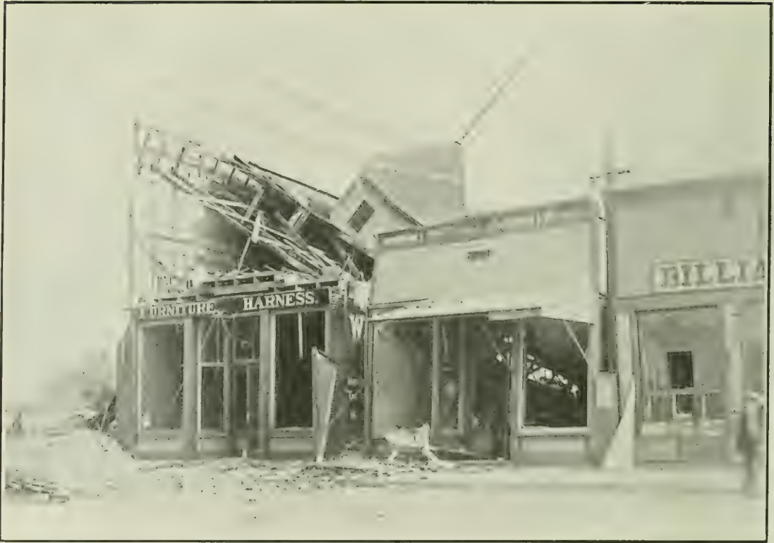
FIG. 11. A PHOTOGRAPH TAKEN IN THE BUSINESS DISTRICT OF SAN JACINTO, CALIFORNIA, FOLLOWING THE EARTHQUAKE OF APRIL 21, 1918. The center building was the telephone office. Note the difference in the damage sustained by the brick and the frame buildings here shown. (Photograph by S. D. Townley.)
