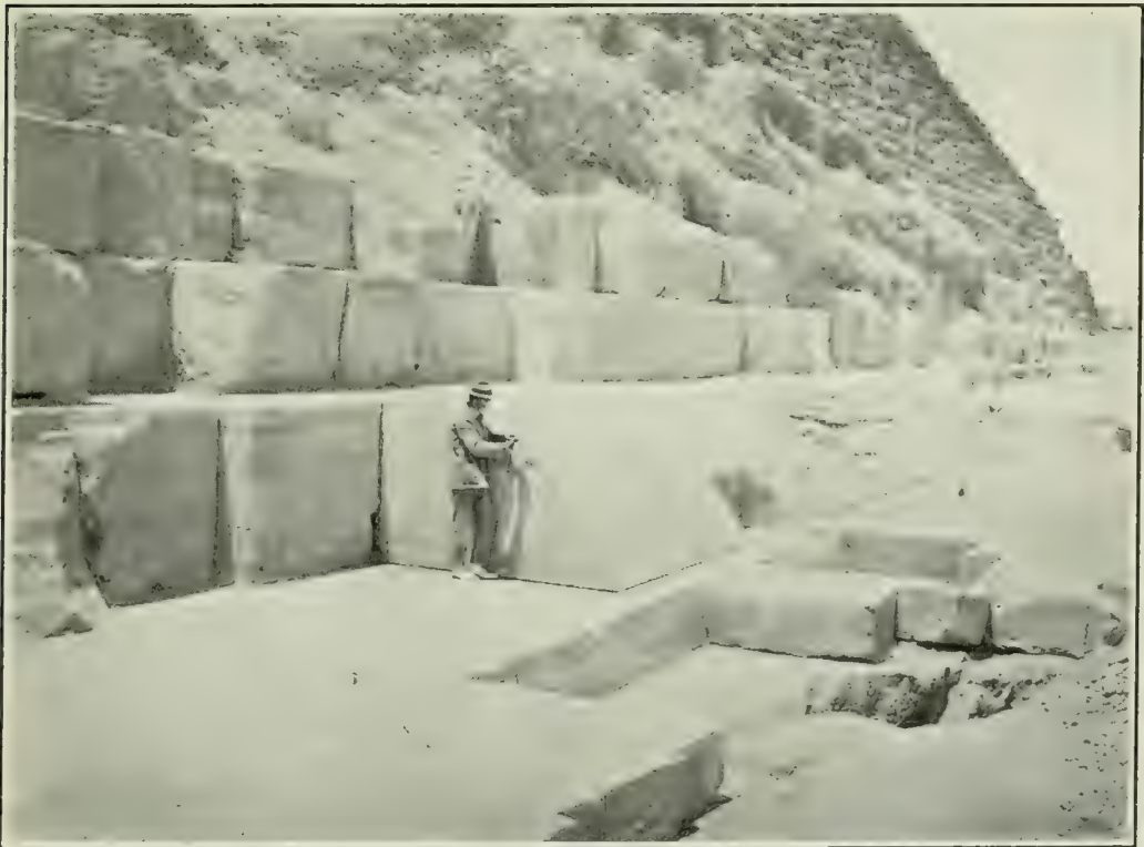
FIG. 72. BLOCKS OF CASING MASONRY OF THE LOWEST COURSE STILL IN POSITION ON THE NORTH SIDE OF THE GREAT PYRAMID. (Photograph by L. Dow Covington.)
