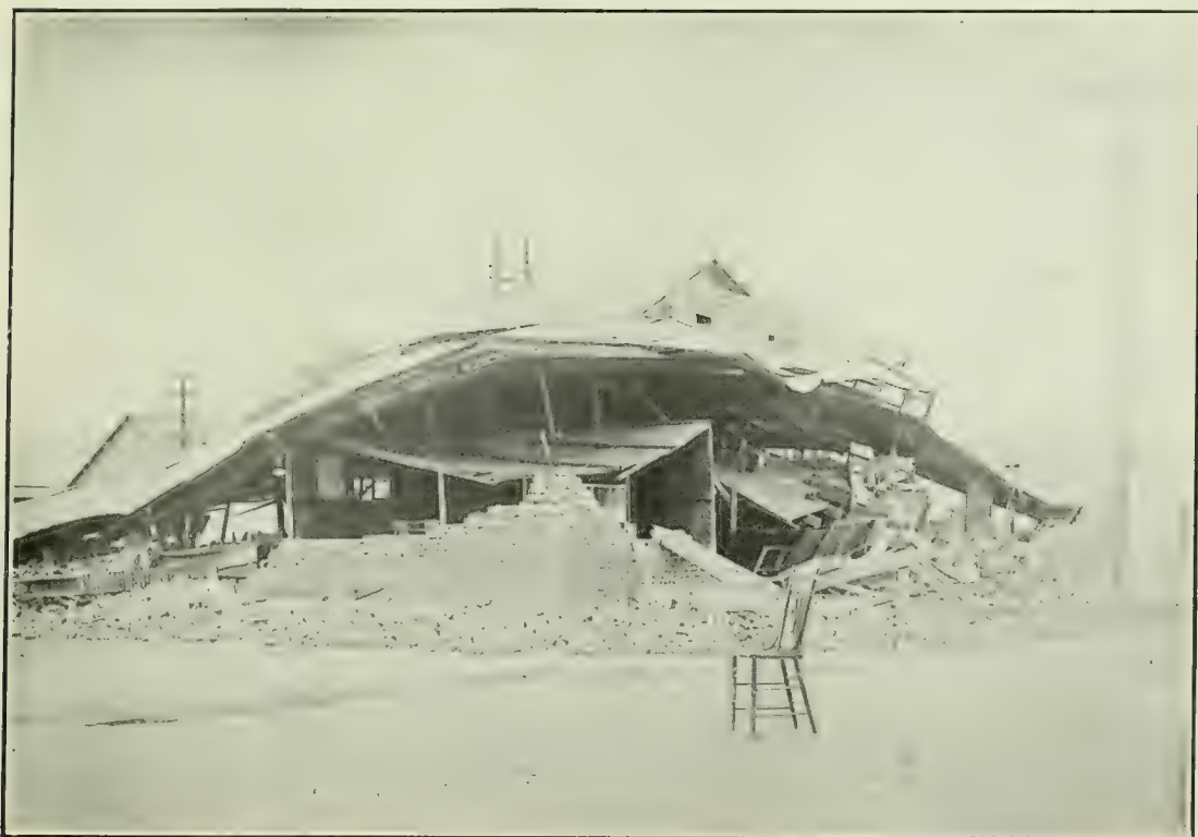
FIG. 2. AN EXAMPLE OF THE DAMAGE SUSTAINED BY BRICK BUILDINGS IN AN EARTHQUAKE. The reinforced concrete building shown in the right background was comparatively unharmed. (Photograph by S. D. Townley.)
