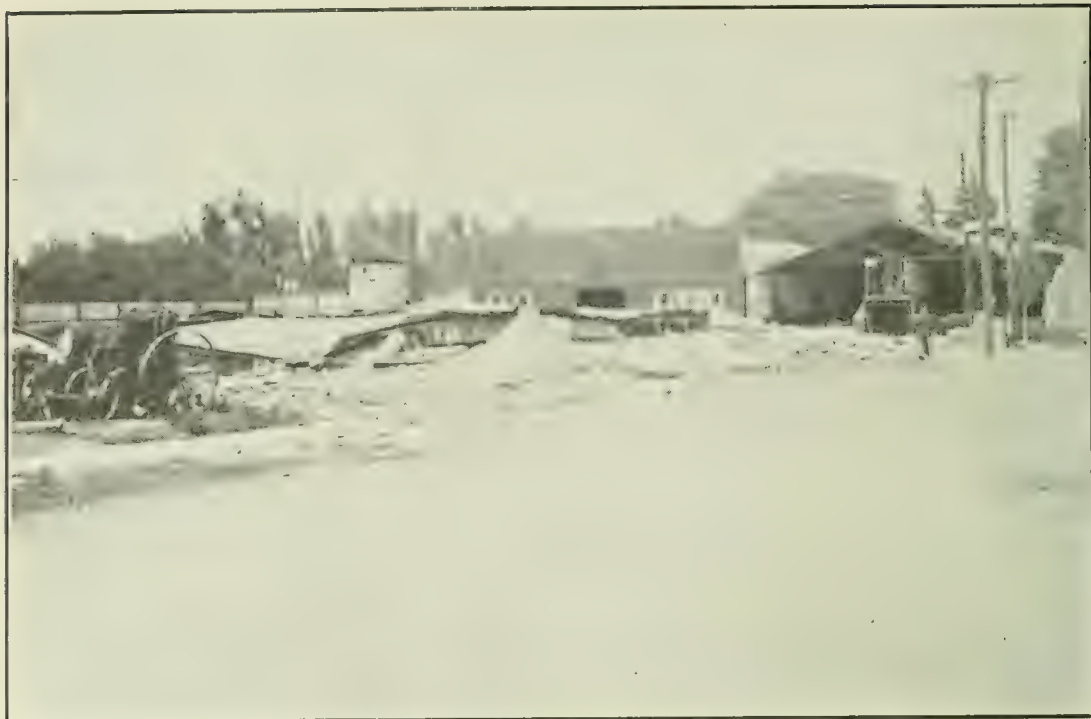
FIG. 7. BUSINESS HOUSES IN SOUTHERN CALIFORNIA LEVELLED TO THE GROUND IN A SEVERE EARTHQUAKE, WHICH CAUSED A PROPERTY LOSS ESTIMATED AT $300,000. (Photograph by Homer Hamlin.)
