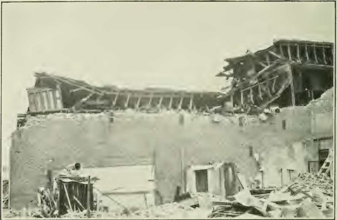
FIG. 9. MASONIC HALL AT SAN JACINTO, CALIFORNIA, wrecked in the Earthquake of April 21, 1918. Note the piano under the roof at the left. Brick buildings can not withstand severe earthquakes. (Photograph by Homer Hamlin.)
