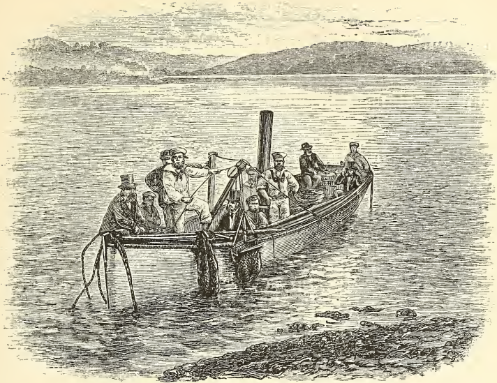
DREDGING ON THE PARAMATTA RIVER, SYDNEY.
