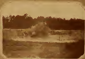
Blasting the site for the Kenan Stadium.
