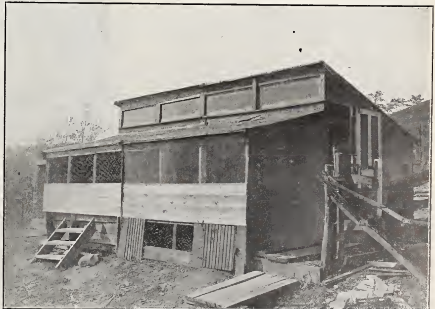
The above is a two section semi-monitor-top open-air poultry house from plans by Dr. Woods as built by J. Frank Parr, East Liverpool, Ohio. It is 20 ft. wide by 16 ft. deep and has a middle partition making it a two pen house. Each pen accommodates thirty-five to forty Black Minorcas. The left pen has an earth floor in front and tight board floor for rear ten feet. The right pen has an entire floor of tight boards with room for a pen below. See plan of open-air house in November A. P. W.—Ed.
