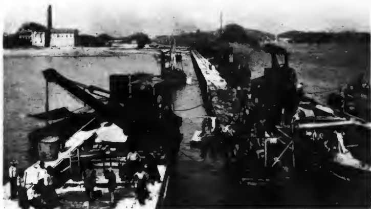
THREE PHASES OF PORT CONSTRUCTION AT RIO DE JANEIRO, BRAZIL.
