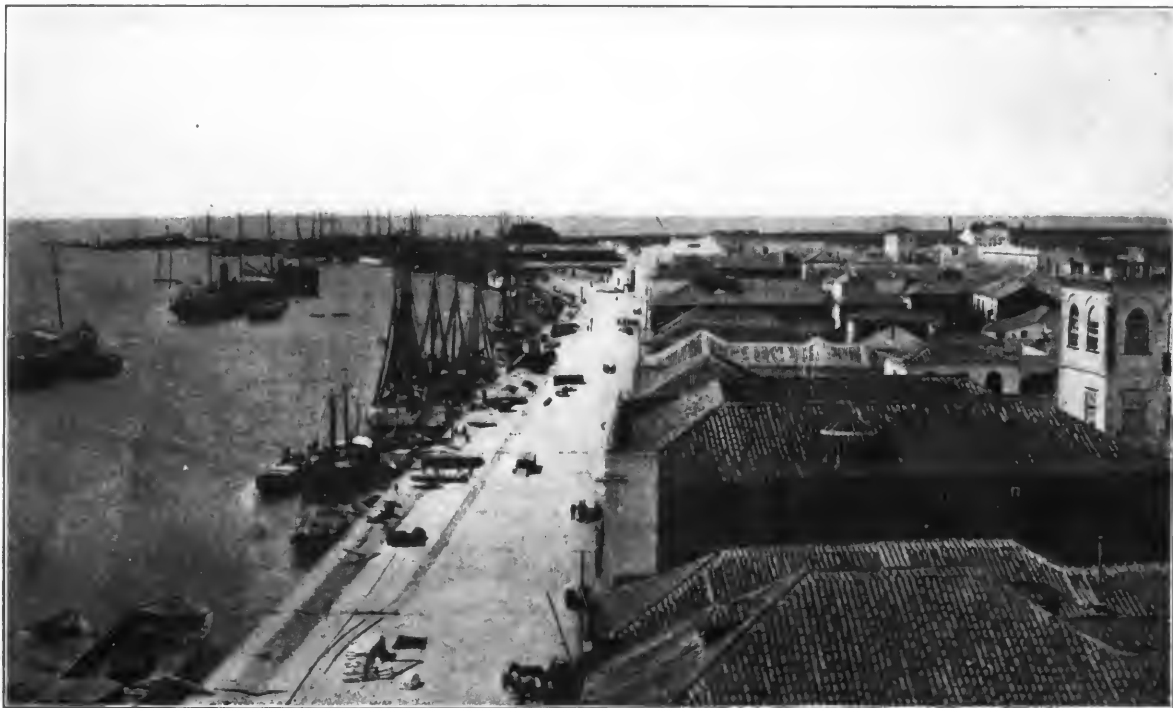
A SECTION OF THE NEW WATER FRONT AT RIO GRANDE DO SUL, BRAZIL.
