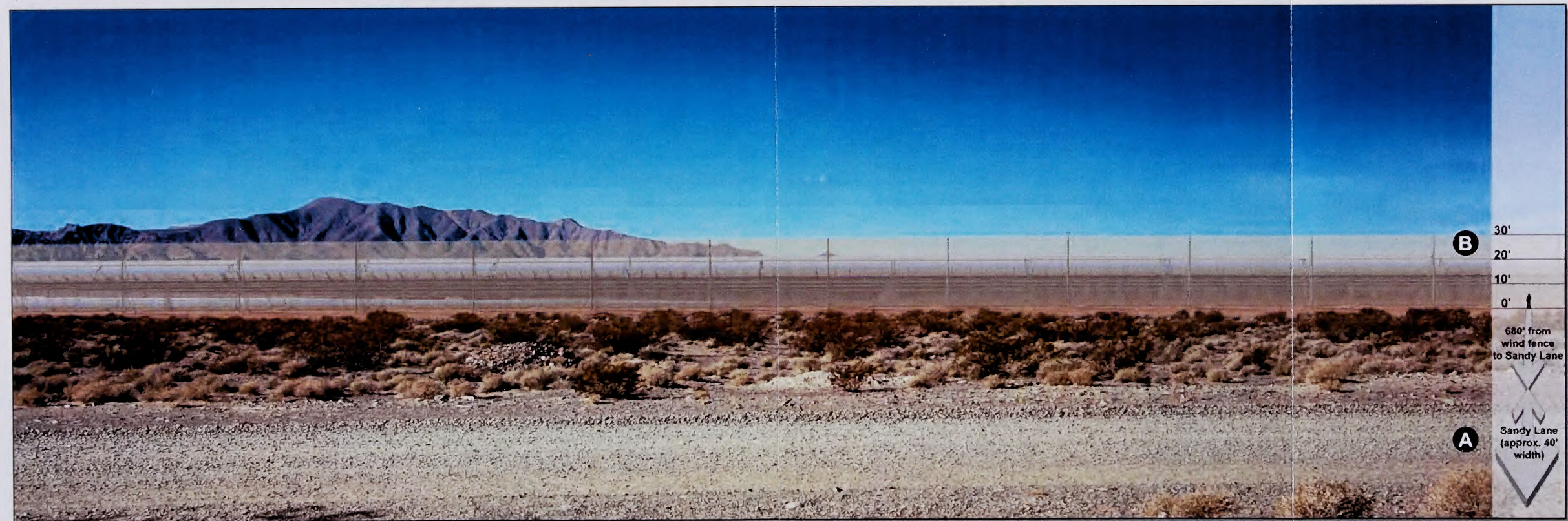
Simulated Condition – Proposed perimeter channel (screened by vegetation), wind fence (30 feet tall), solar fields, and thermal energy storage tanks
