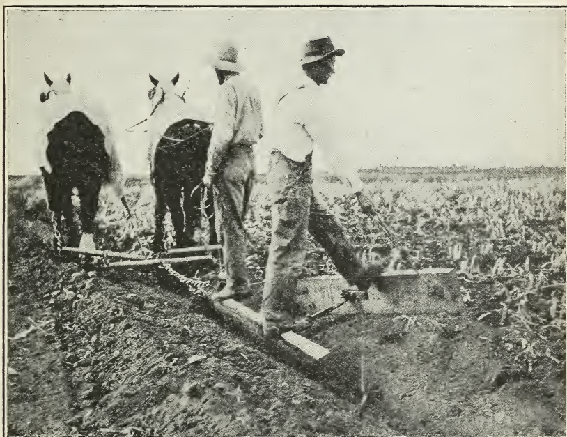
FIG. 15.—Constructing an irrigation ditch on the Belle Fourche Experiment Farm. The corn ground is irrigated before sowing it to winter wheat.
