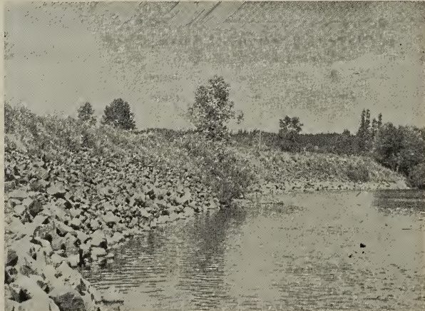
Rock ripraps, brush mats, revetments, jetties, and bulkheads are built along Washington river banks.
