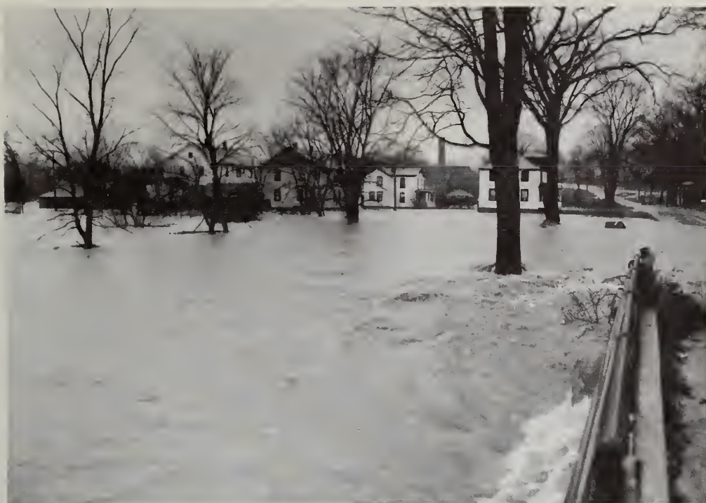
Pittsfield -- Looking westerly along the Cadwell Road Bridge over the Southwest Branch and Zoar Avenue, New Year flood of 1948-1949.
