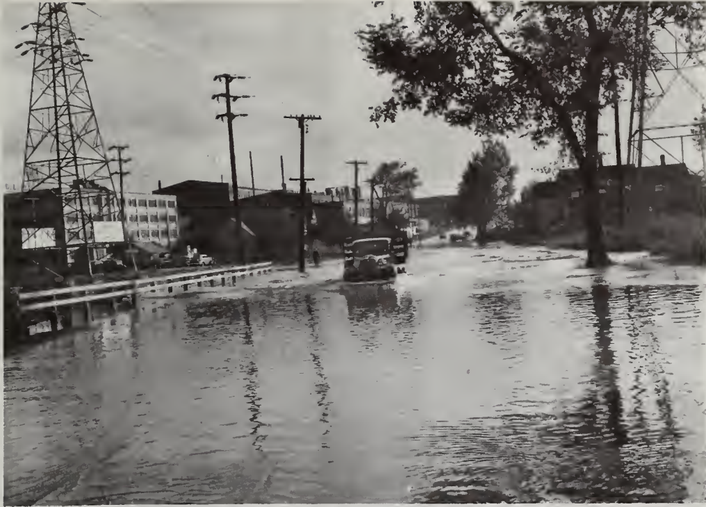
Pittsfield -- Looking northeasterly along East Street in the vicinity of Silver Lake and the East Branch, flood of September 1938.
