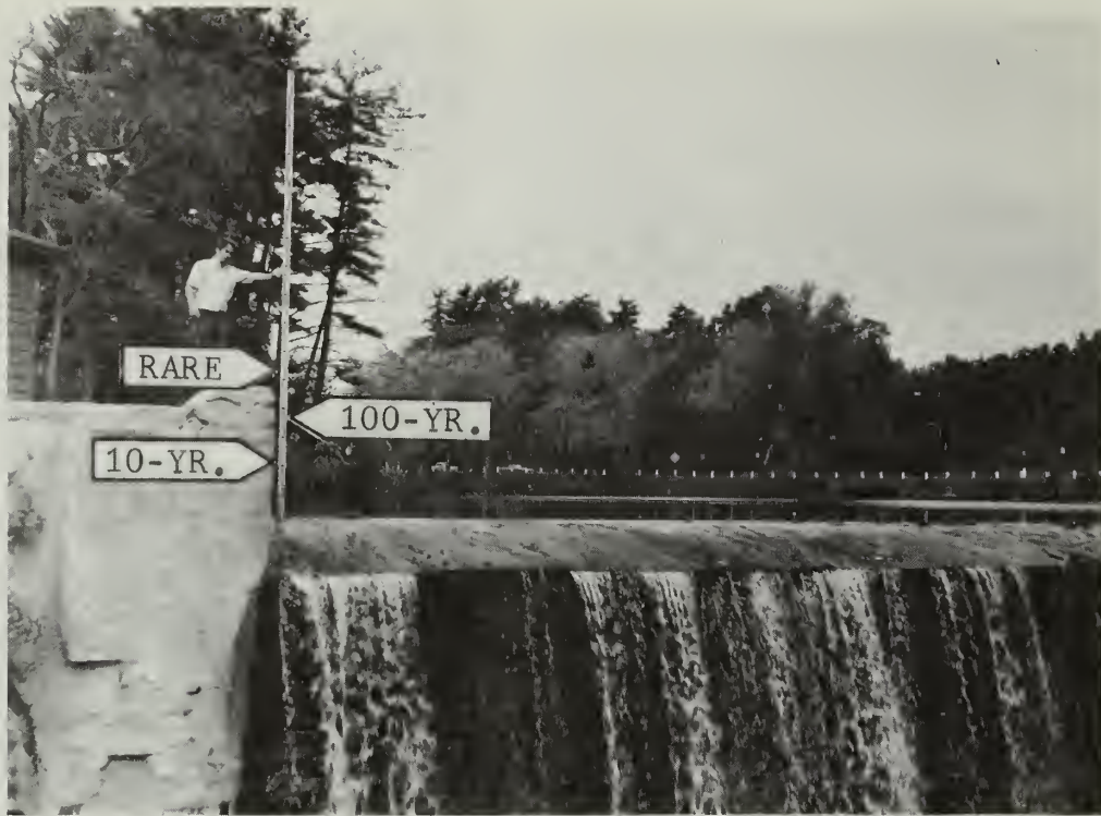
Pittsfield -- Pontoosuc Lake Dam, with U.S. Route 7 in background.
