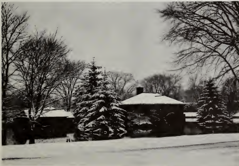
Pomeroy Avenue Pumping Station along East Branch, New Year flood of 1948-1949.
