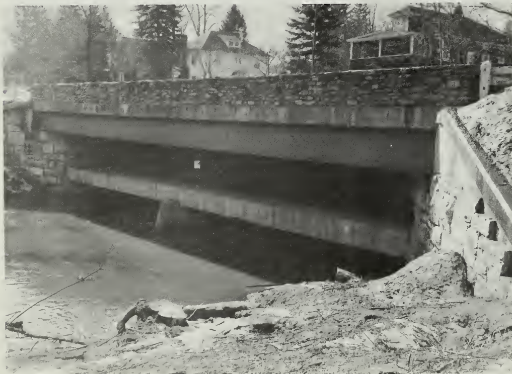
South Street Crossing over the Housatonic River, with utility conduit.
