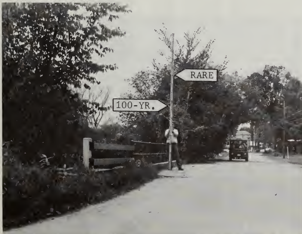
Pittsfield -- Looking westerly at the Cadwell Road Bridge over the Southwest Branch.
