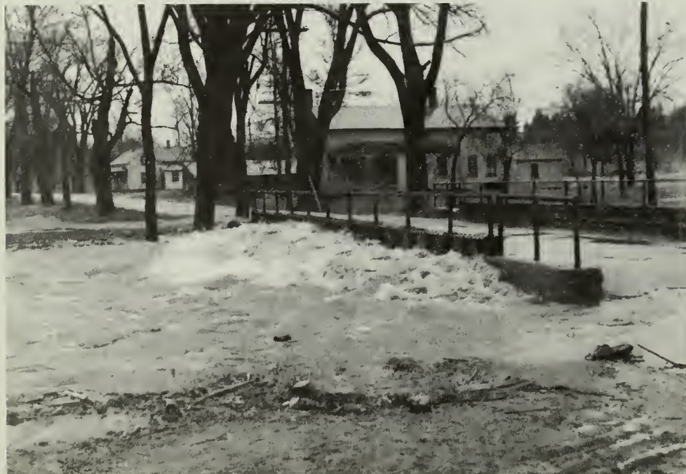
Hubbard Avenue bridge over the East Branch, September 1938 flood.
