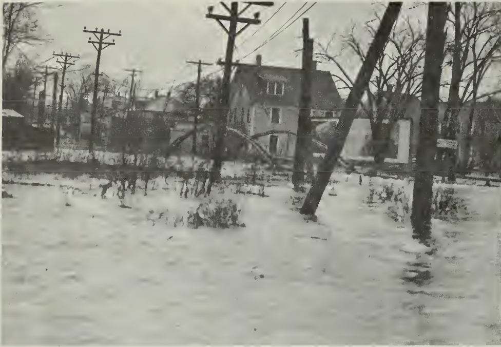
Newell Street bridge over East Branch; September 1938 flood.
